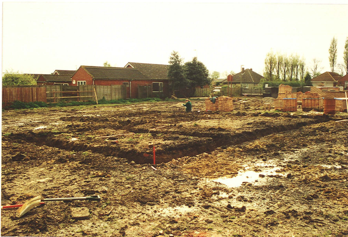
Pl. 1 Site of Plot 1, looking south.
