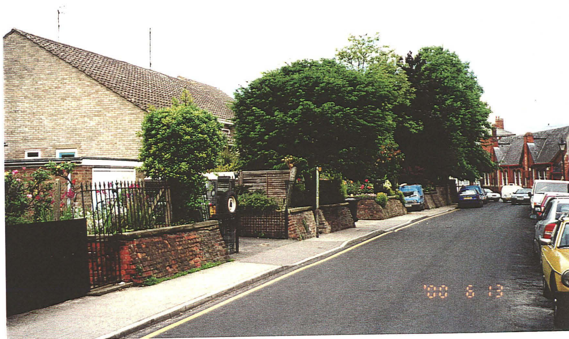
Plate 5: Witham Place looking west. Note the battered brick walls retaining each of the raised gardens created when the tidal salt marsh was reclaimed. The iron railings and gates are also an original feature.
