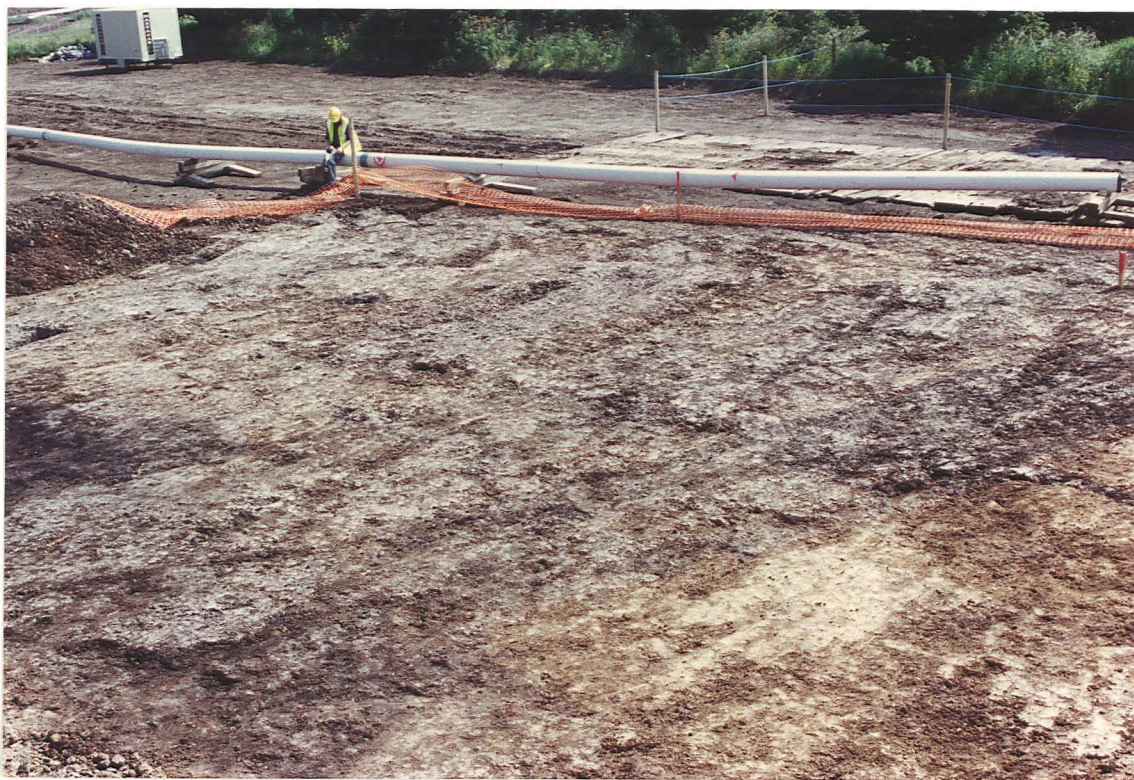
Pl. 21 Excavation Area B, Field 17, prior to excavation (looking SW).
