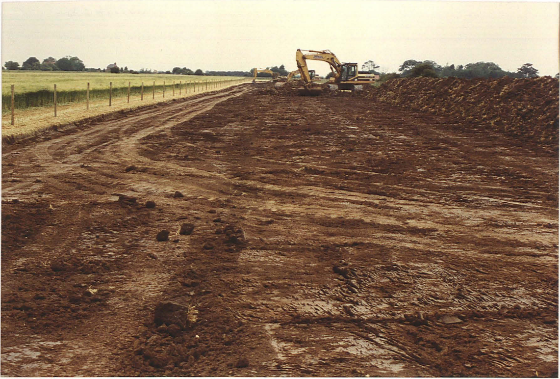
Pl. 1 Topsoil stripping in progress, Field 27 (looking NW).
