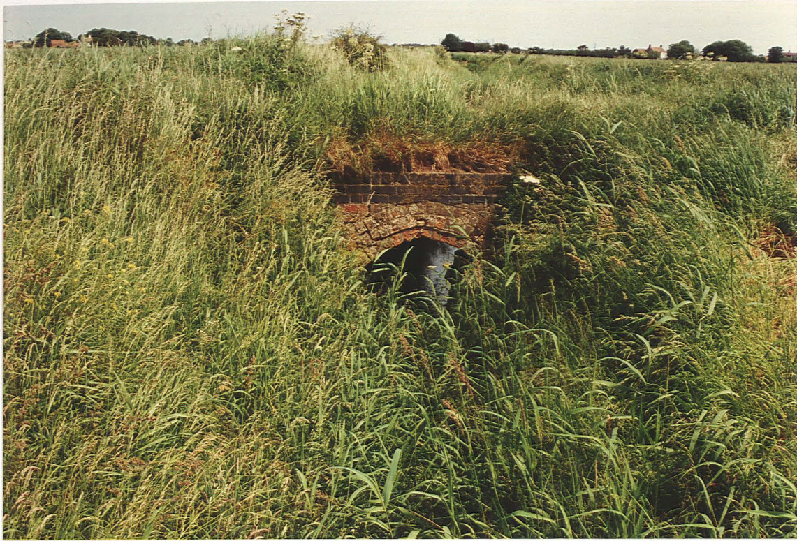
Pl. 7 Engineering bricks in the bridge formerly carrying the railway track over field drainage ditches between Fields 12 and 13. Looking east.
