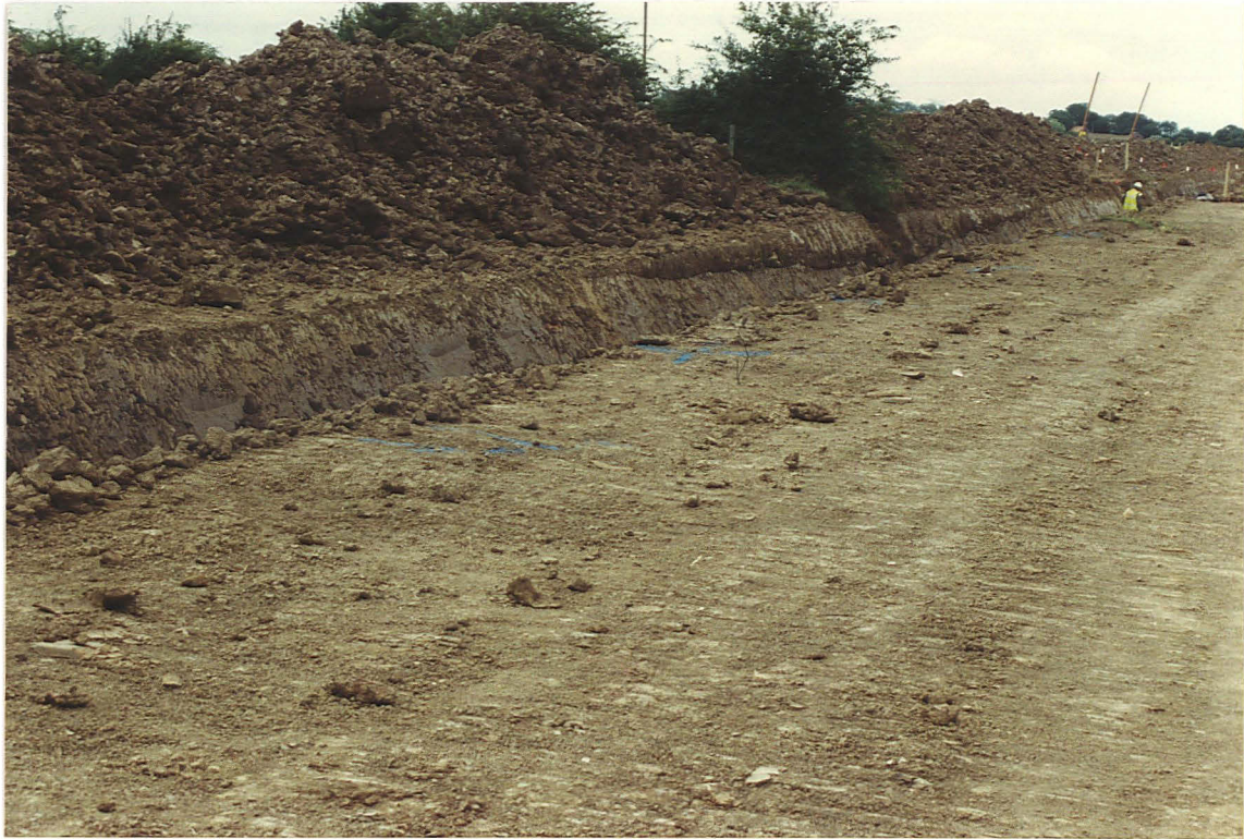
PI. 3 Peat layer covered by silt visible in the pipe trench face, marking a broad depression between Fields 7 and 8. Looking west.
