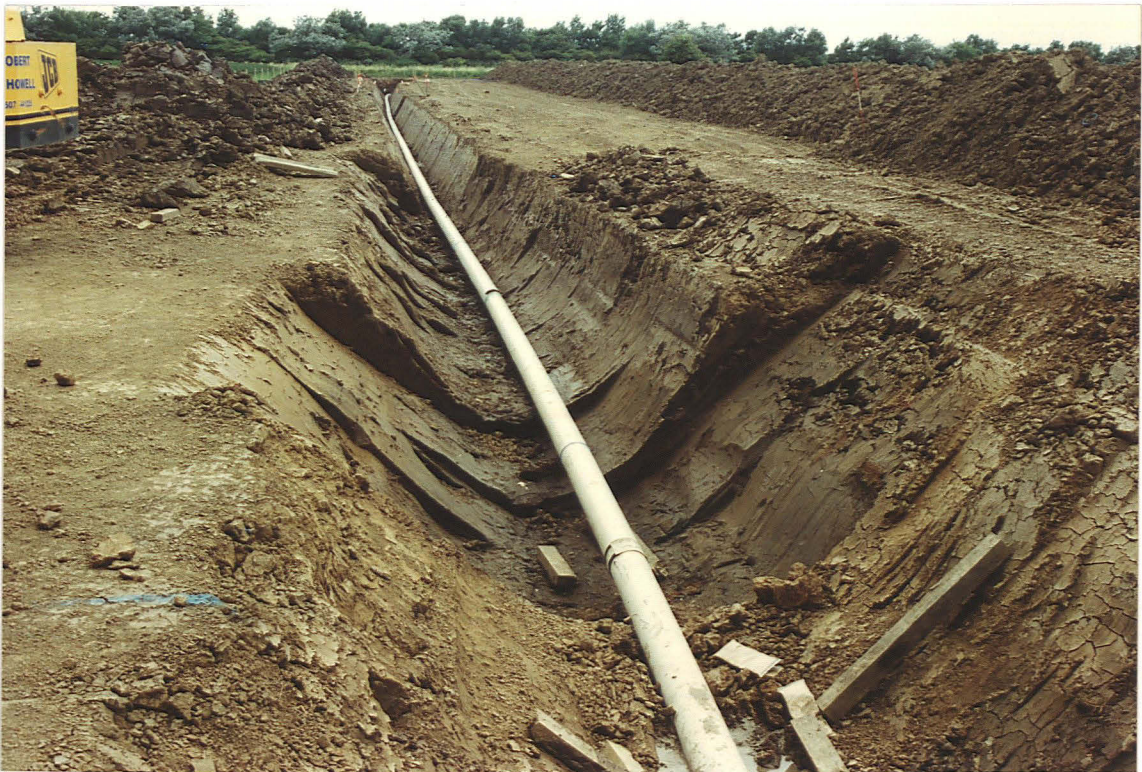
Pl. 2 The pipe trench after excavation, Field 4.
