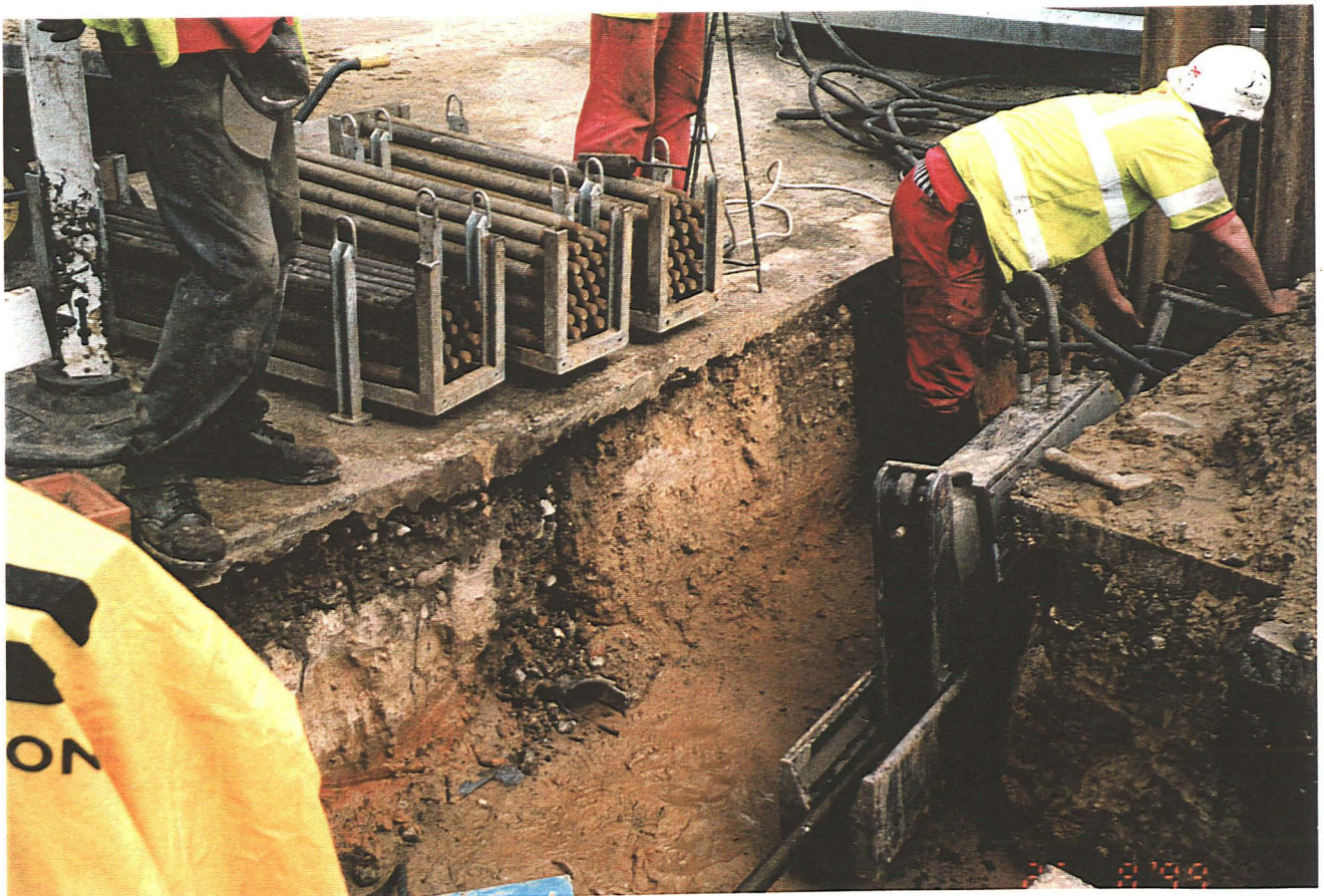
P4. Access trench at junction of North Street/Church Street
