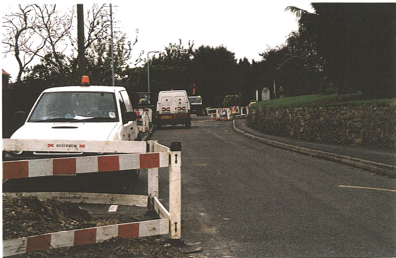
P1. Access pits on Church Street, looking west
