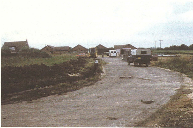
Plate 1 General view of site
