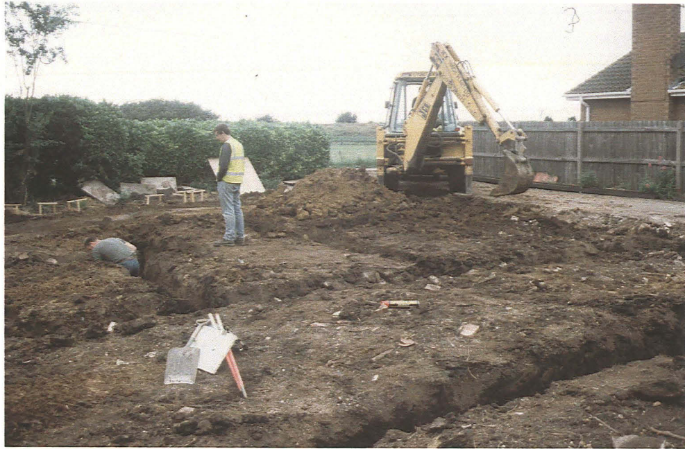
Plate 1 General view of the excavated foundation Trenches, looking north
