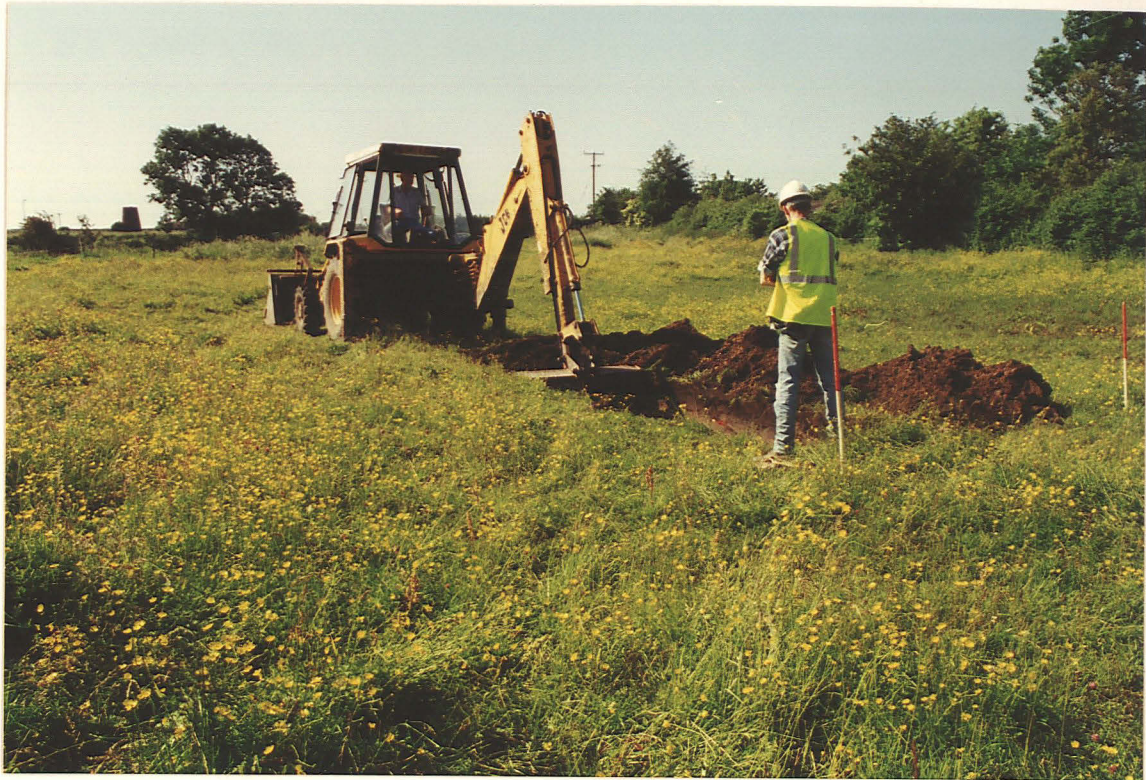
Pl. 1 Machine excavation of trenches under archaeological supervision.
