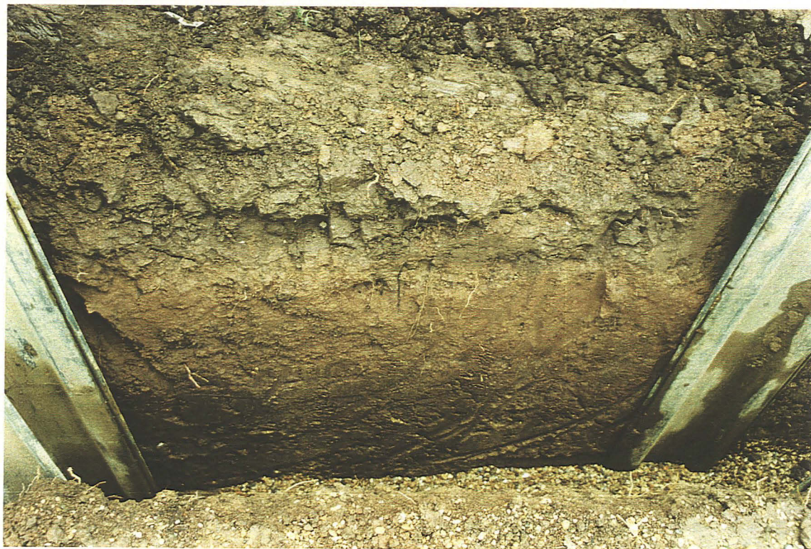
Plate 2: Excavation of storm drain, illustrating soils present on the site
