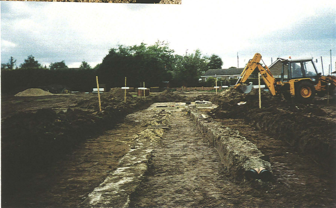
Plate 4: Excavation of the roadway, facing west
