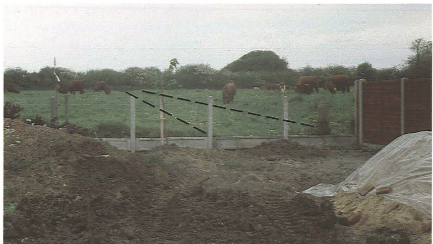
Plate 3 General view of earthwork ditch/channel to the northwest of site, looking north
