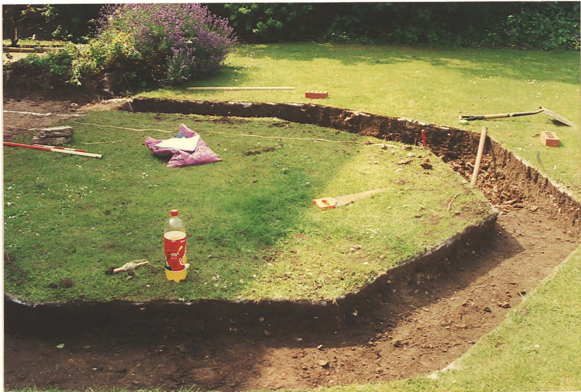
Pl. 2 Partially excavated foundation trenches for the conservatory, looking south
