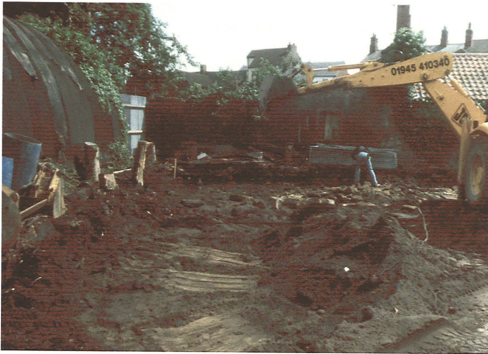
Plate 1 - General view of the development area during site operations, looking south
