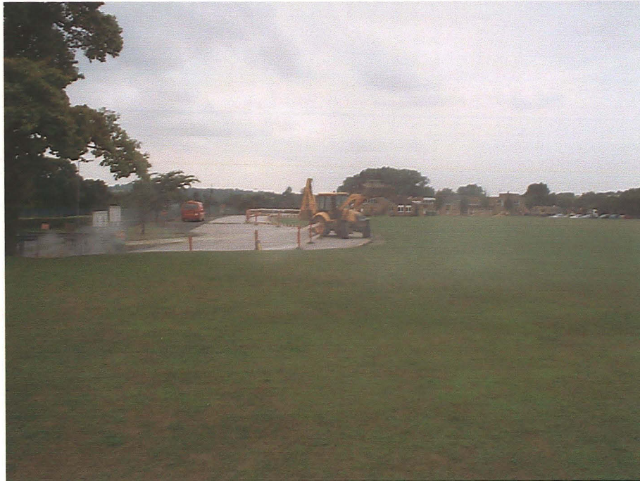
Plate 5 General view of route of gas pipeline, looking northwest
