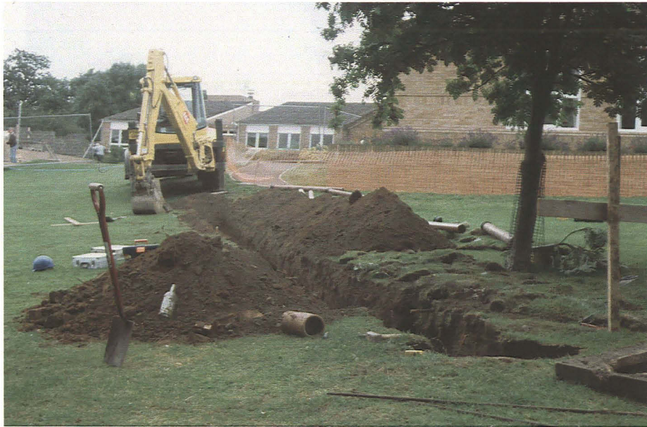
Plate 3 General shot of service trench, looking northeast towards the school
