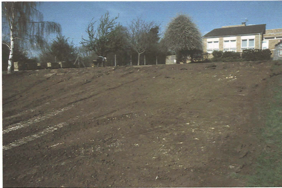
Plate 1 General view of topsoil stripping, looking northeast towards the school
