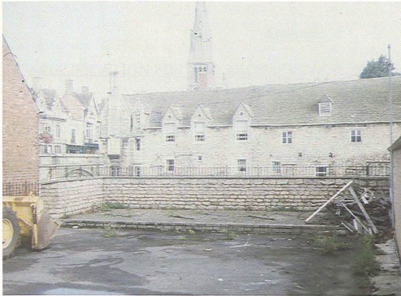
Plate 1 - General view of the development area, looking north
