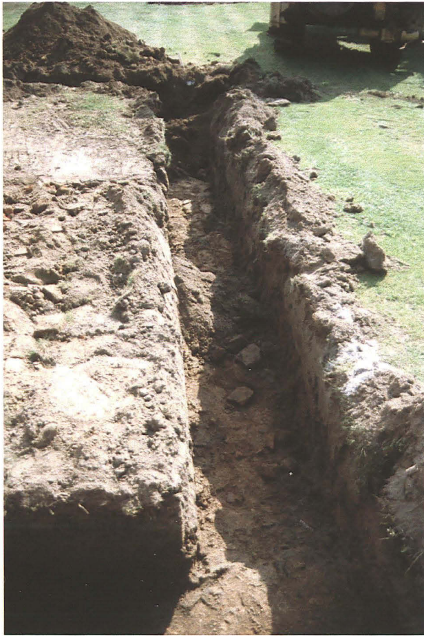
◀ Plate 1 General view of the foundation trenches looking southwest
