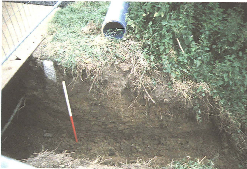
Plate 2 View of road embankment, Section 2, looking south
