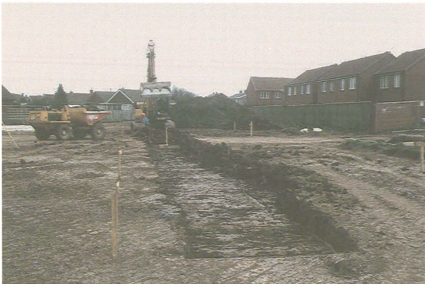
Plate 2 General view of the road stripping in progress, looking southeast
