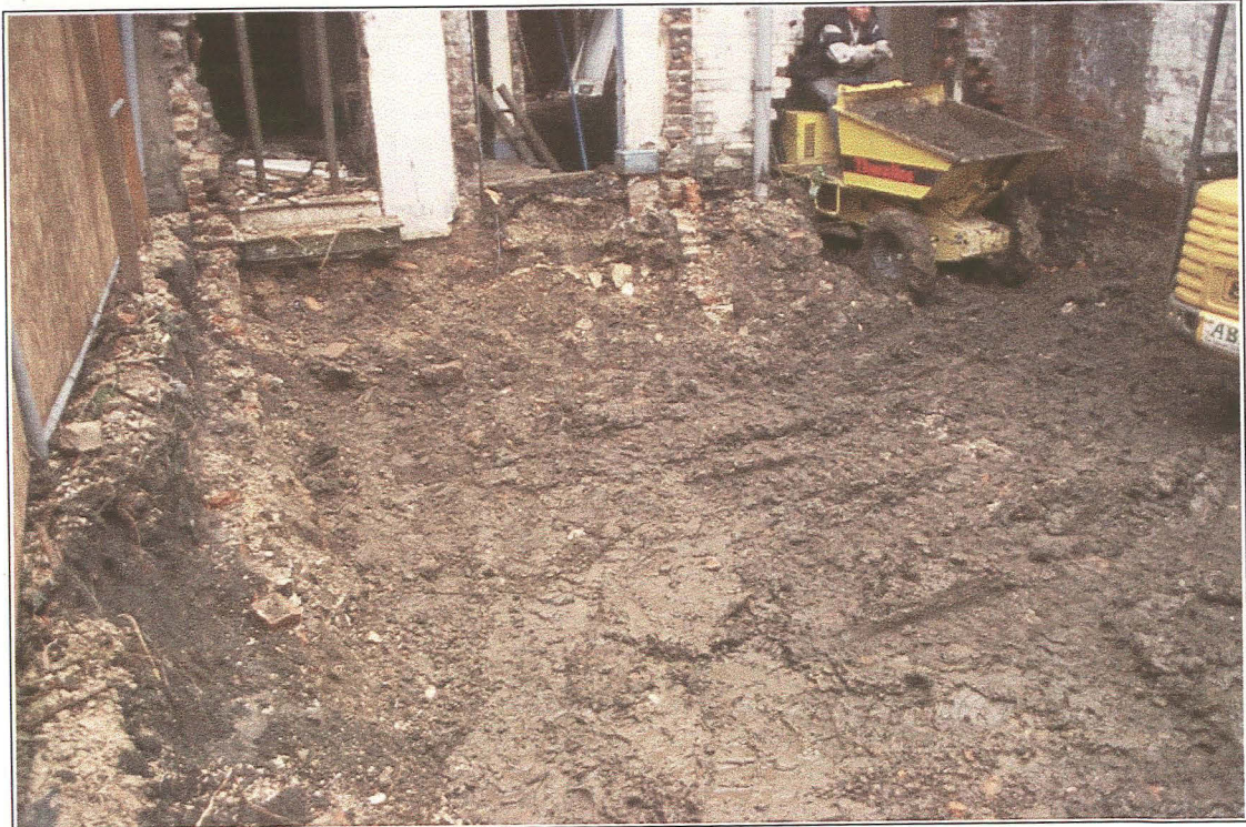
Plate 1 - General view of stripped rear yard (looking east).
