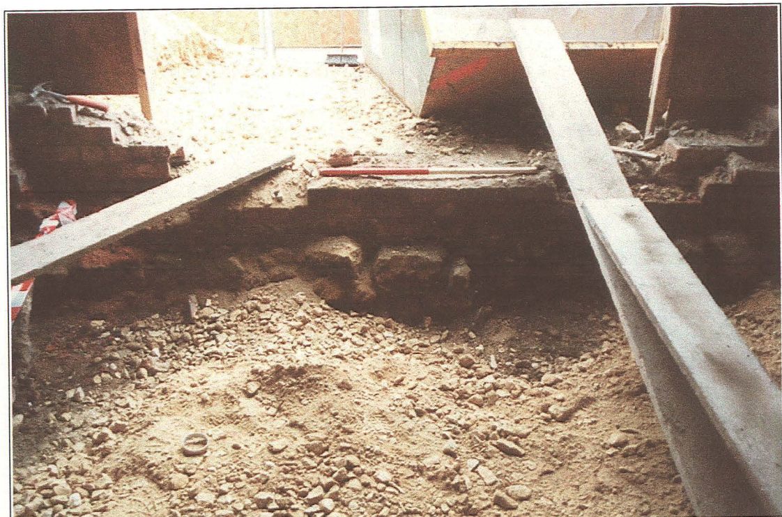
Plate 2 - General view of limestone foundations along the shop frontage (looking east).
