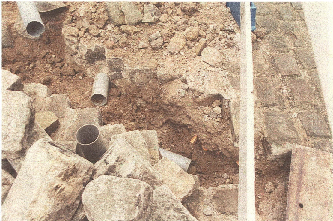
Plate 2: Overall view of excavated section - looking north
