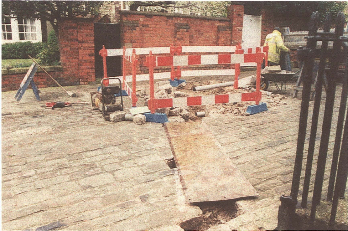
Plate 1: General view of trench across Minster Yard - looking north-west
