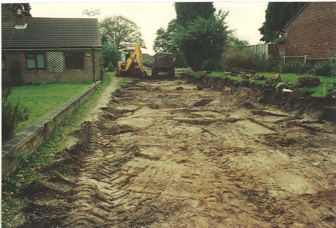
PI. 2 Access road following topsoil stripping.
