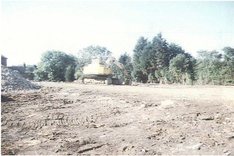
Plate 1 General view during excavation
