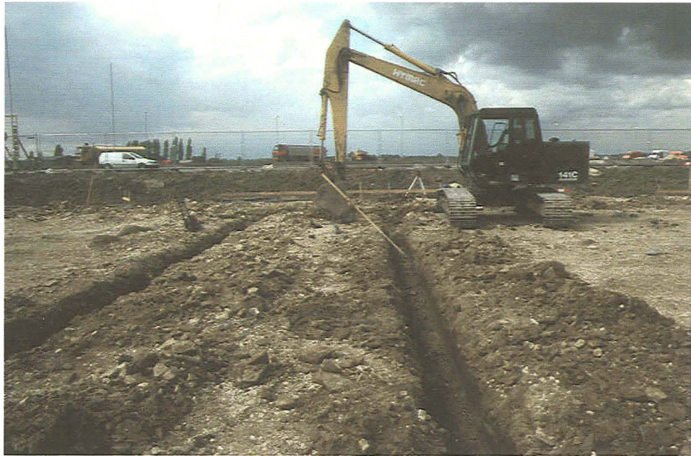
Plate 1 General view of site during groundworks
