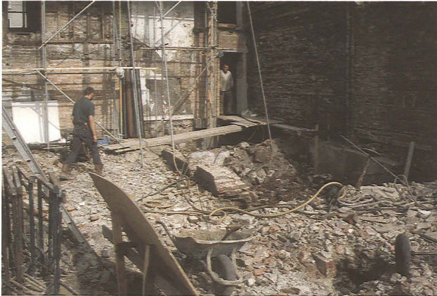
Plate 1 General view of site, looking west
