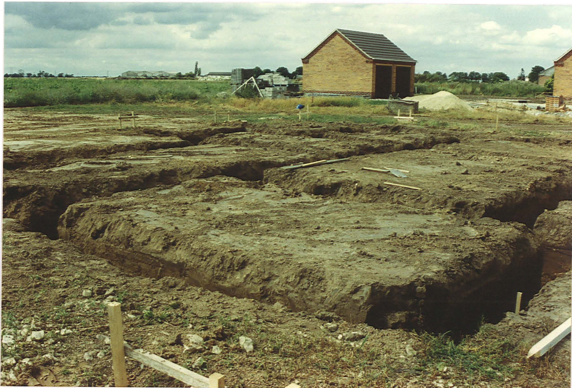
Pl. 6 Foundation trenches for Plot 4 (looking NW towards the garage for Plot 6).
