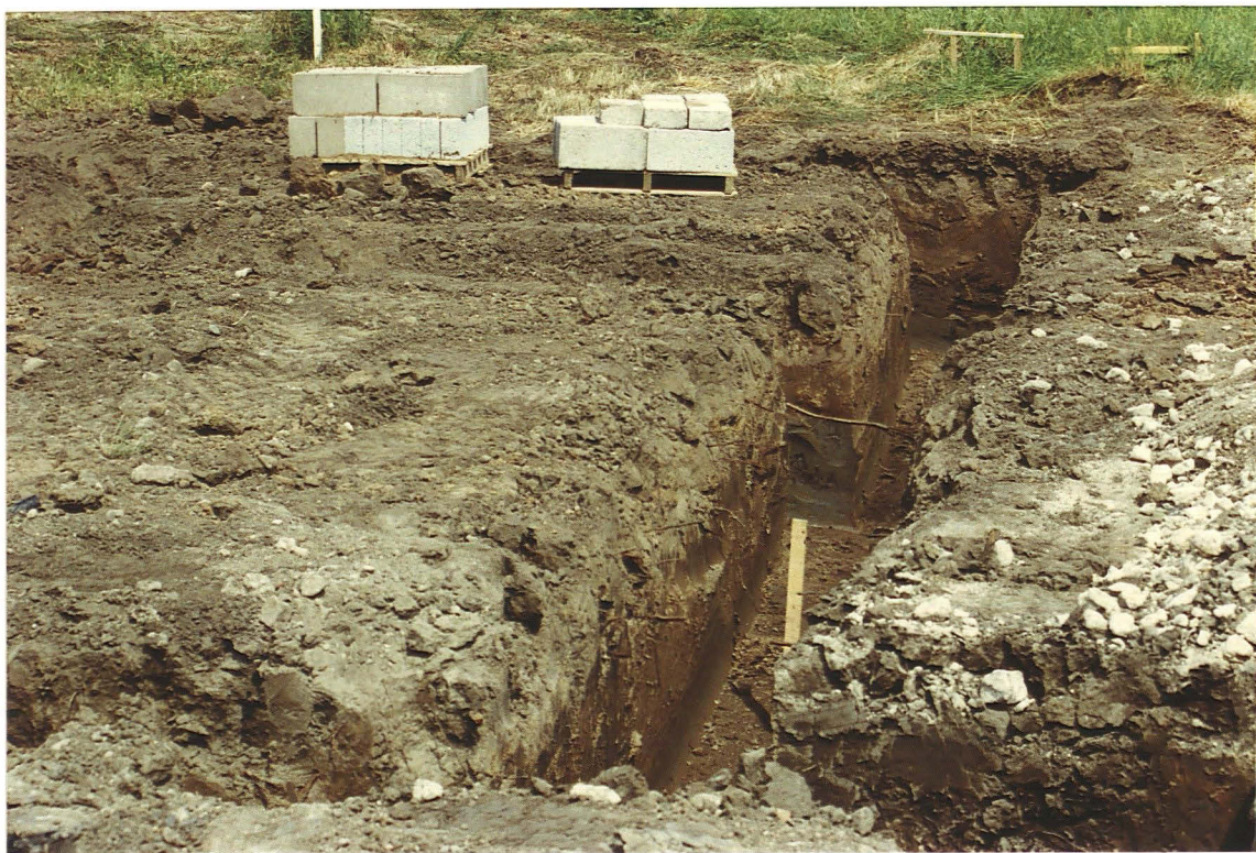
Pl. 4 Silt deposits in the trench face at C (looking west).
