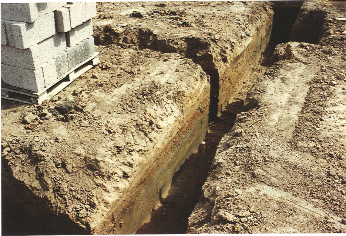
Pl. 3 Silt deposits at B, close to Friest Lane (looking east).
