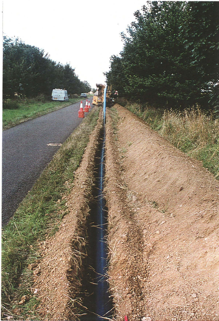
Plate 1: Working shot, showing simultaneous trenching and pipe laying (looking west).
