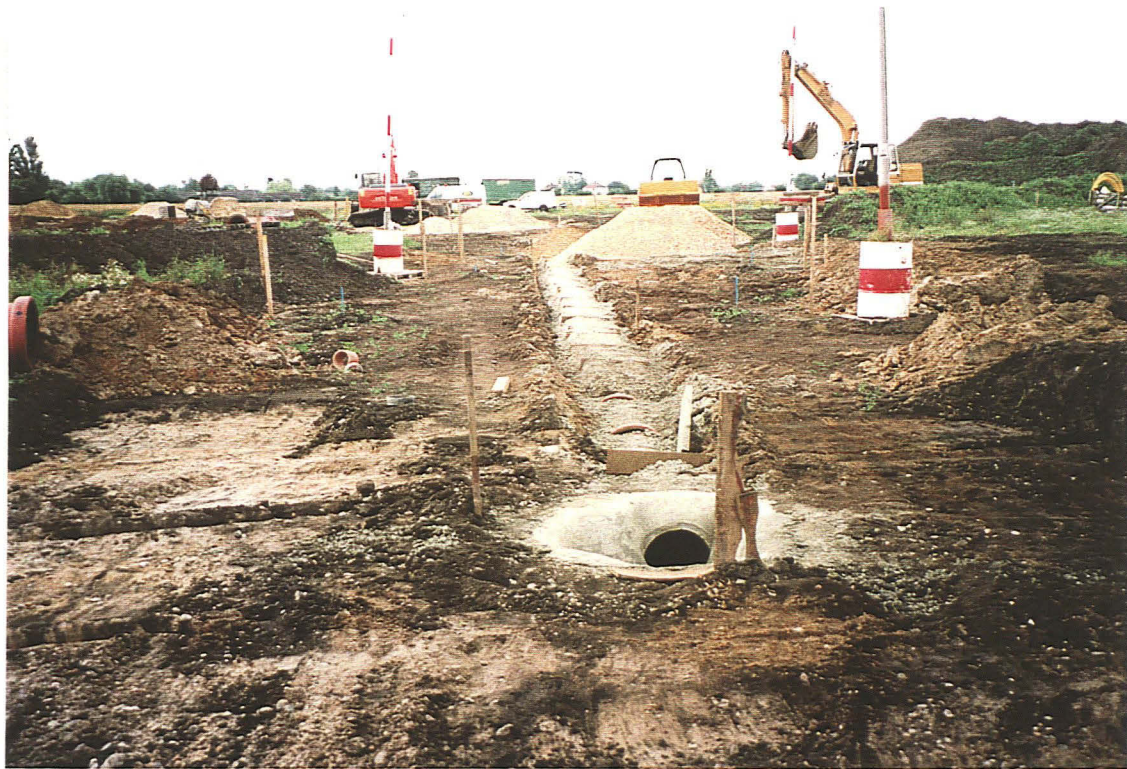
P4. Phase I area, central access and sewer construction, looking north-west
