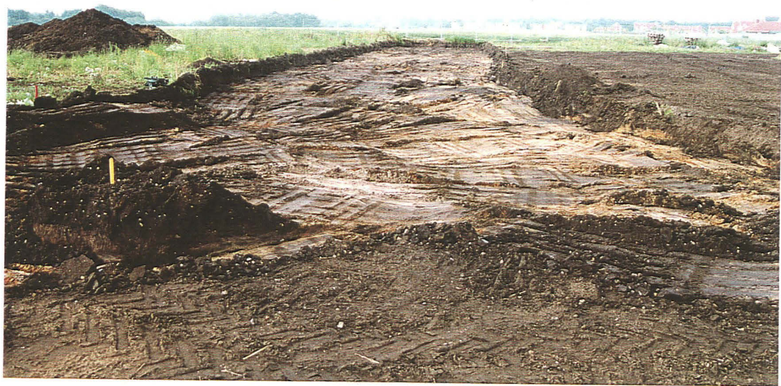
P5. Eastern access, Phase II area, following soil stripping, looking east
