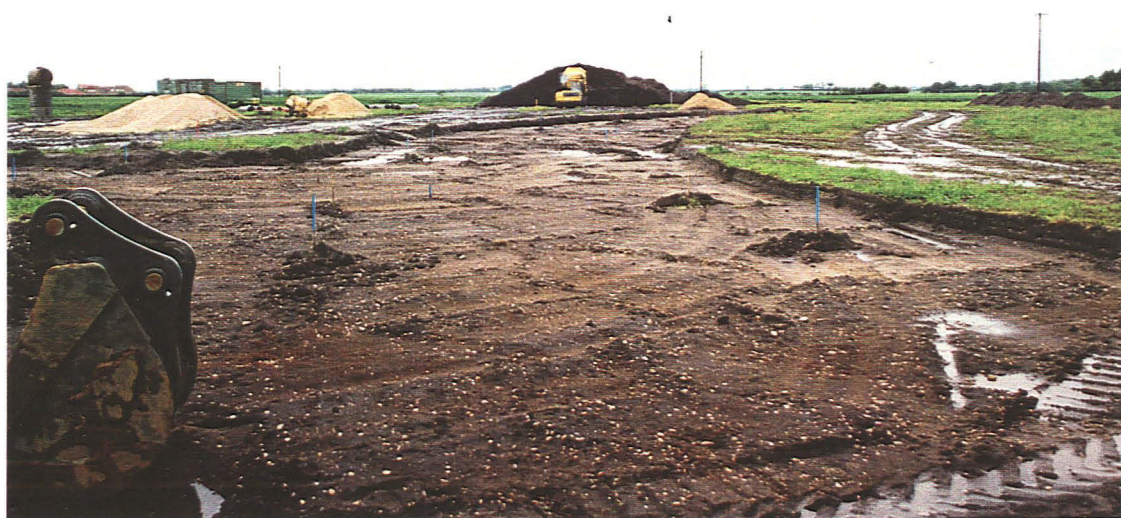
P2. Soil stripping of the southern access (Phase I), looking NNW
