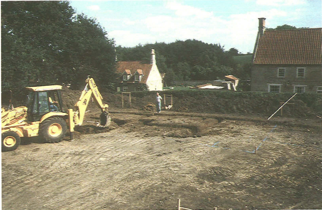
Plate 1 General view of site prior to the groundworks
