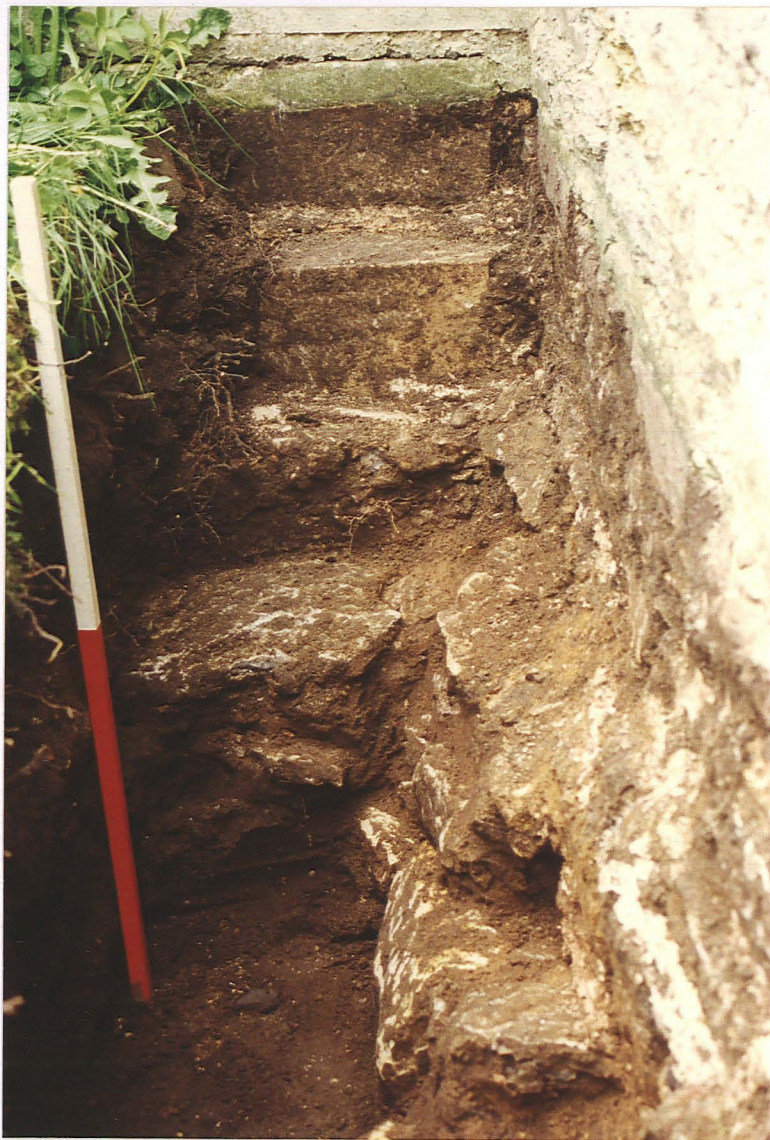
Pl. 18 Detail of porch and south aisle foundations which appear to be contemporary, with two later courses above
