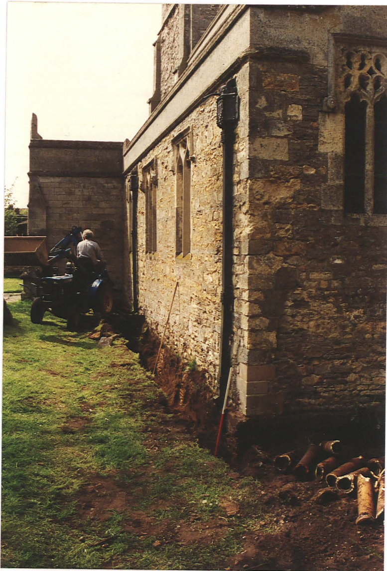
Pl. 14 General view along south aisle south wall
