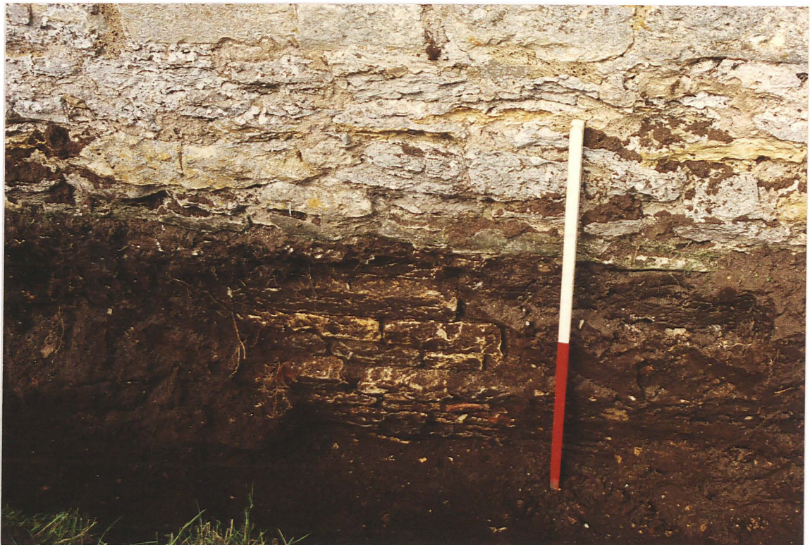
Pl. 15 Detail of south aisle south wall foundations east of the windows
