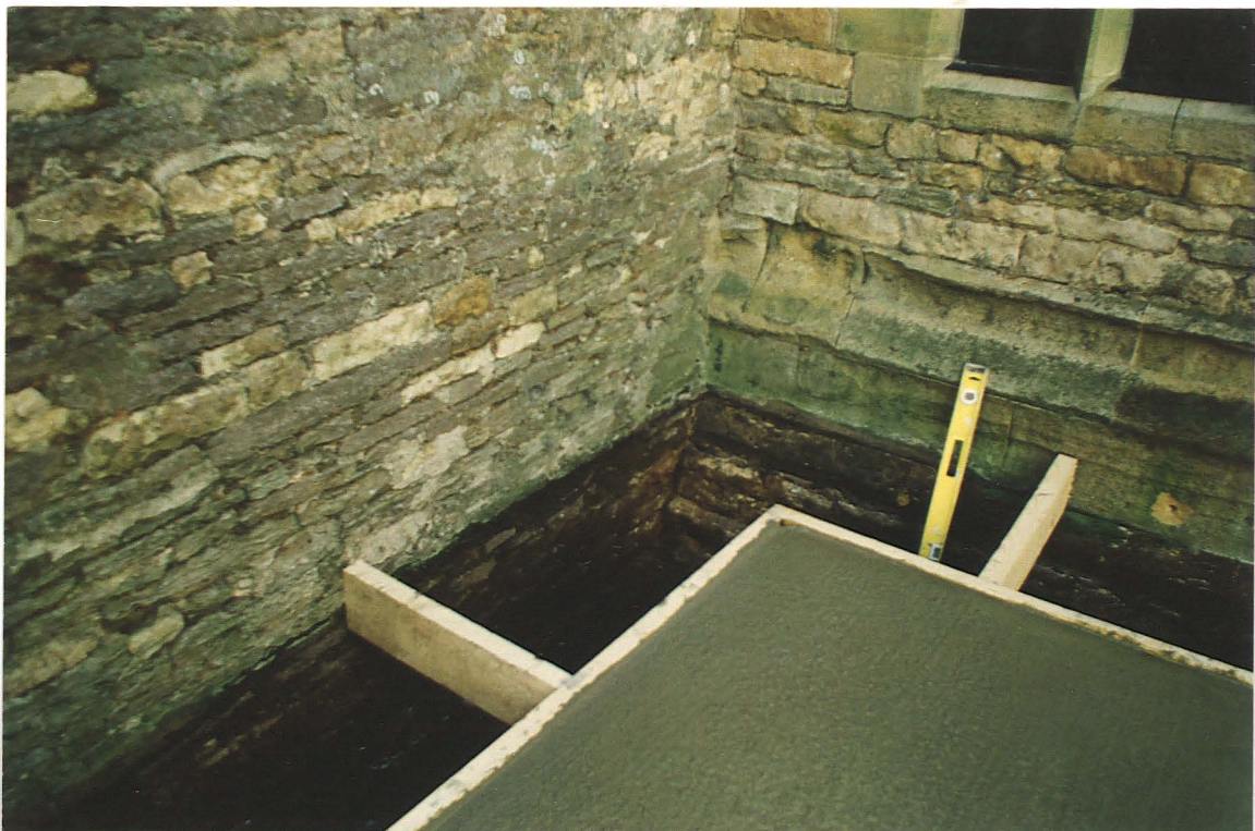
Pl. 13 Detail showing vestry wall (right) butting chancel north wall (right)
