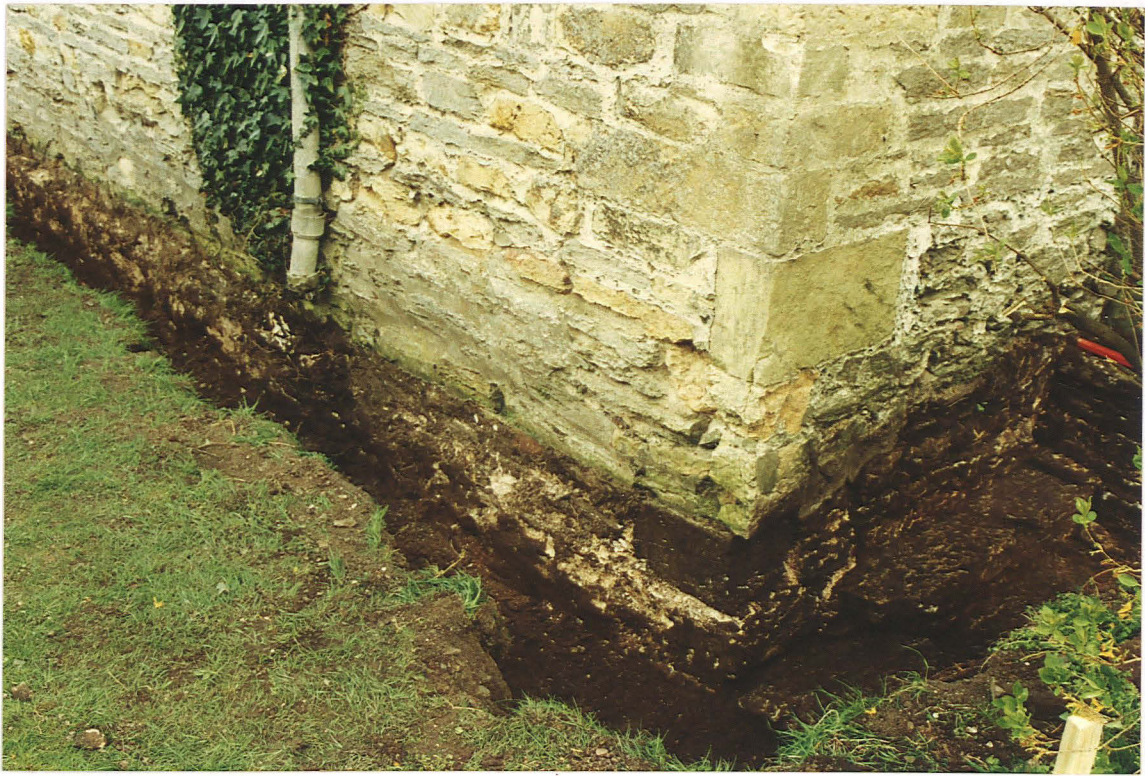
Pl. 8 NW angle of the north aisle showing different character of the foundations along the north and west walls
