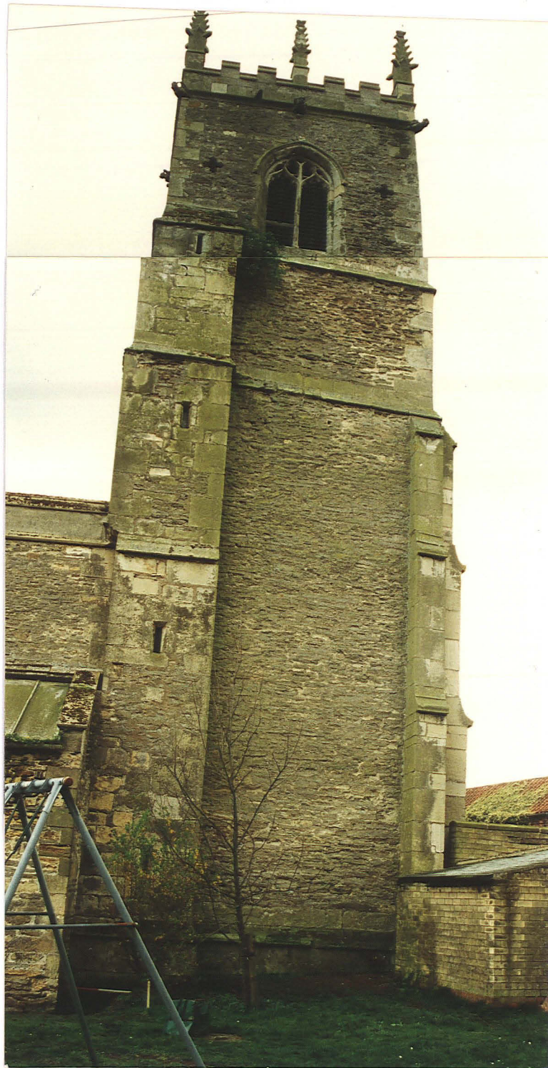
PI. 5 North side of Laughton church tower with stair turret in NE angle
