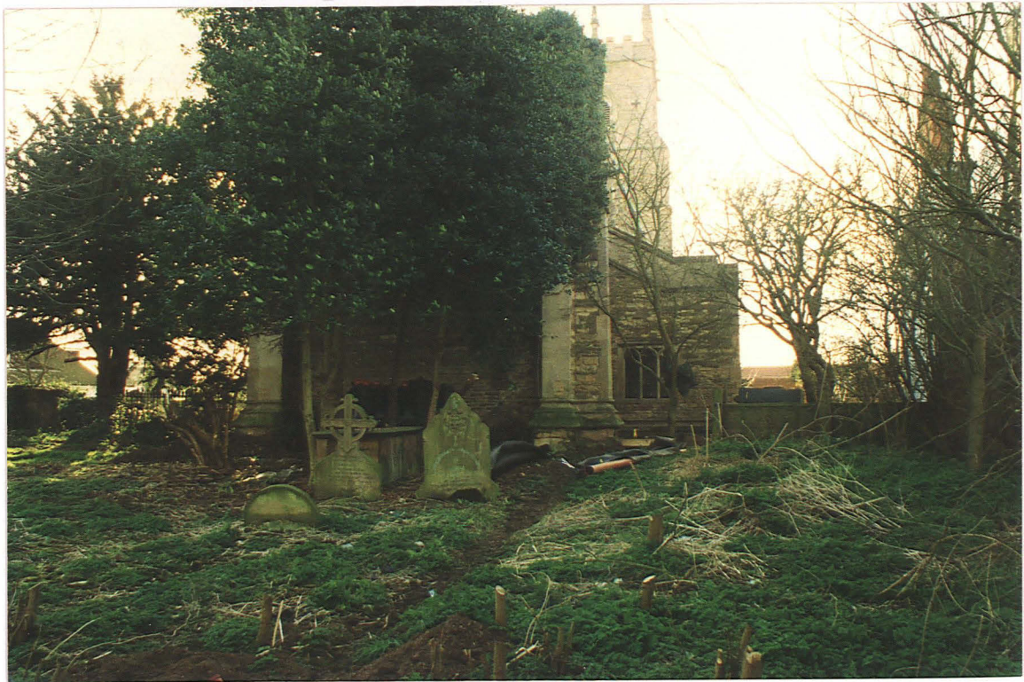
Pl. 11 General view of east end of church showing chancel and vestry
