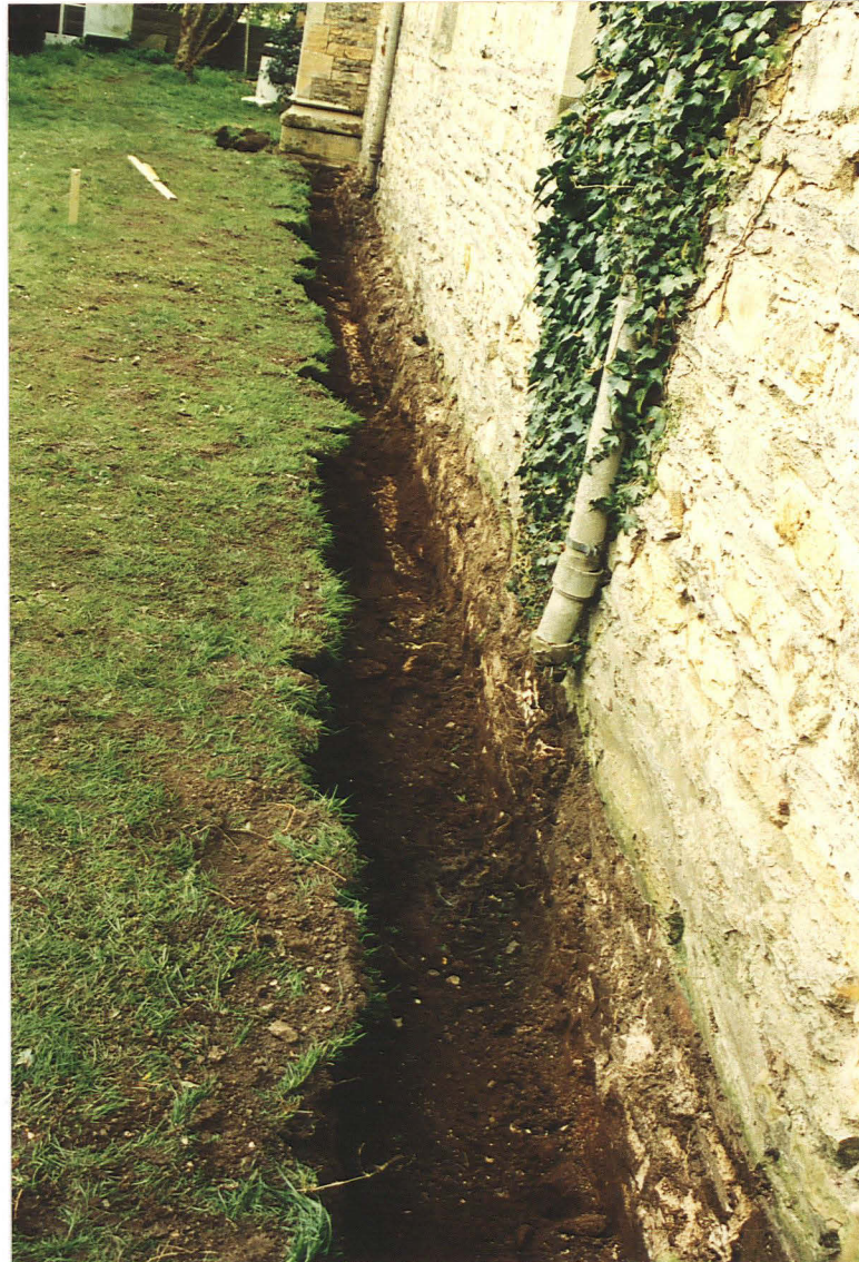
Pl. 9 View looking east along north aisle north wall showing neat, off-set foundations of small sized stone
