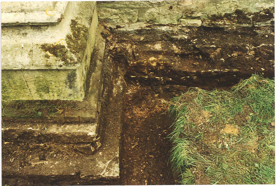
Pl. 10 Added buttress at junction of north aisle and vestry
