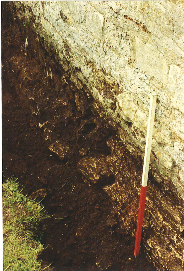
Pl. 16 Junction of rubble and coursed foundations beneath south aisle south wall
