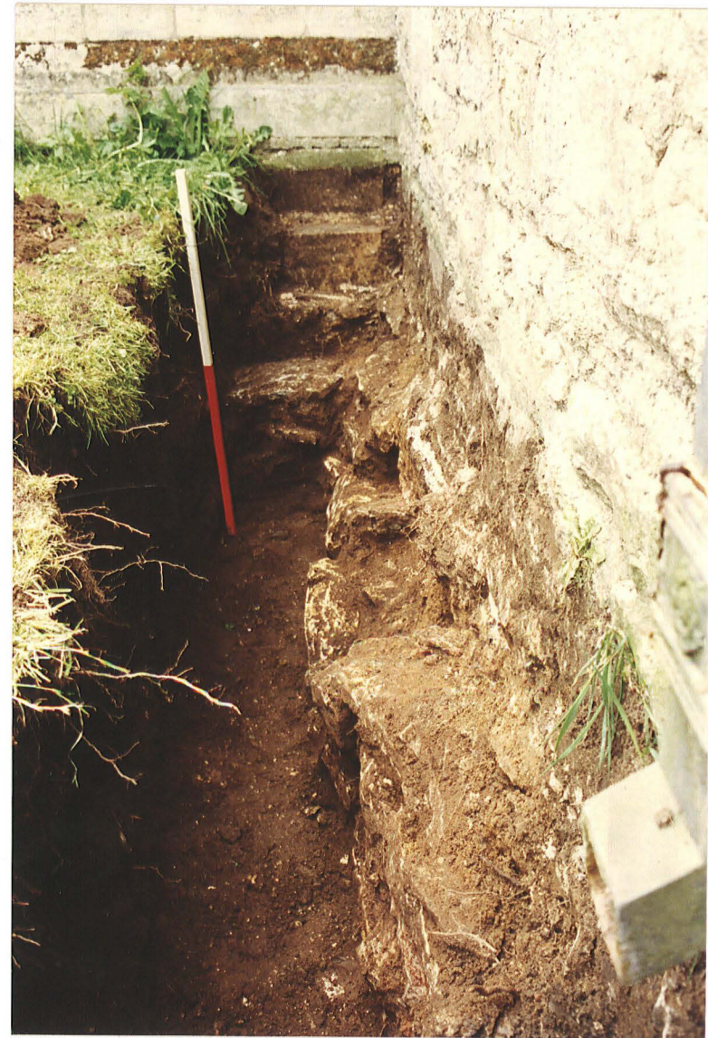
Pl. 16 Junction of rubble and coursed foundations beneath south aisle south wall
