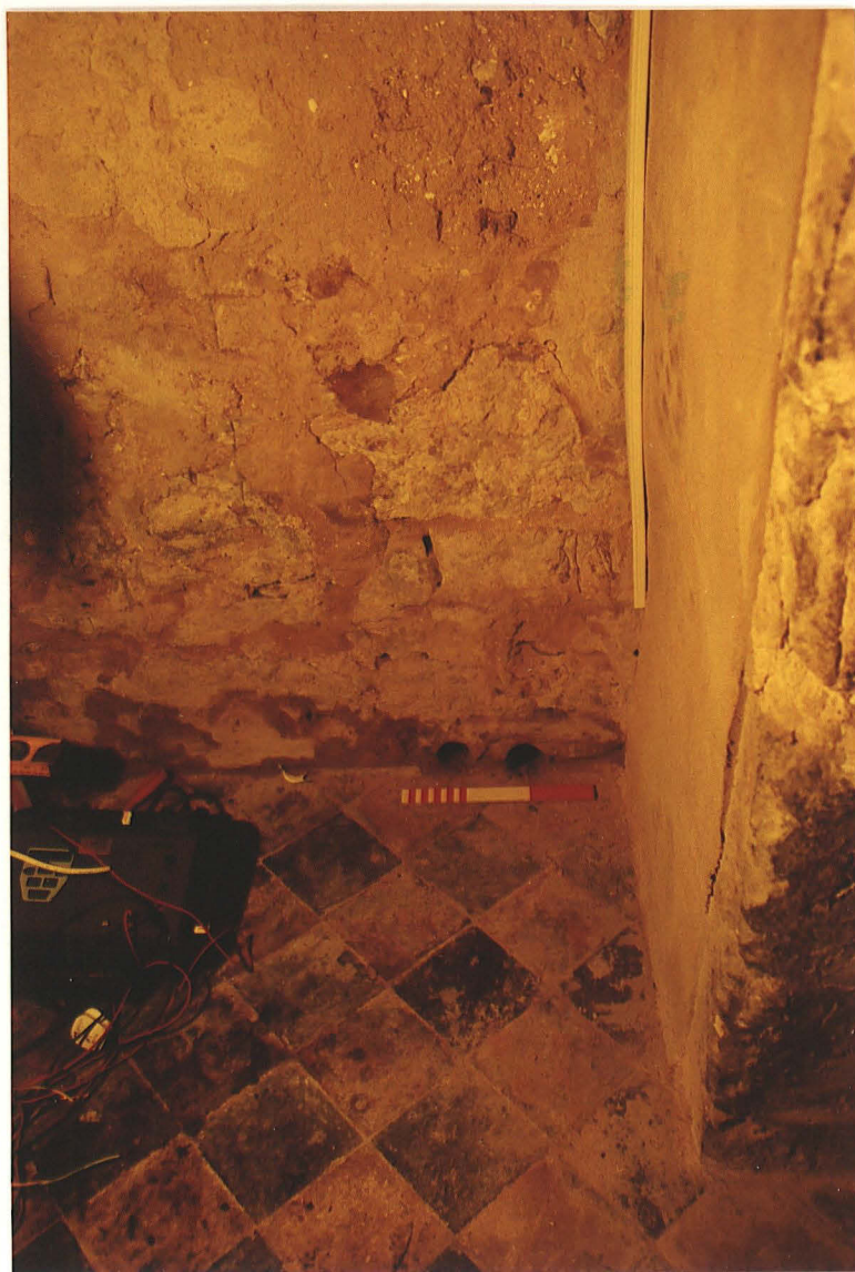
Pl. 5 Two holes drilled through the tower north wall for the new services (interior view, looking north; scale 0.3m).
