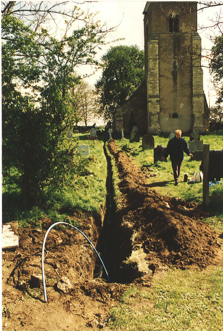
Pl. 3 Service trench with water pipe and cable duct installed (looking east).
