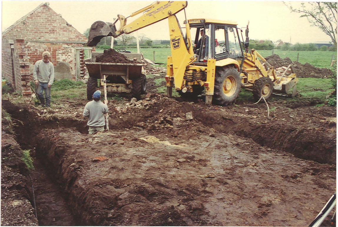
Pl. 5 Excavation of foundations looking east
