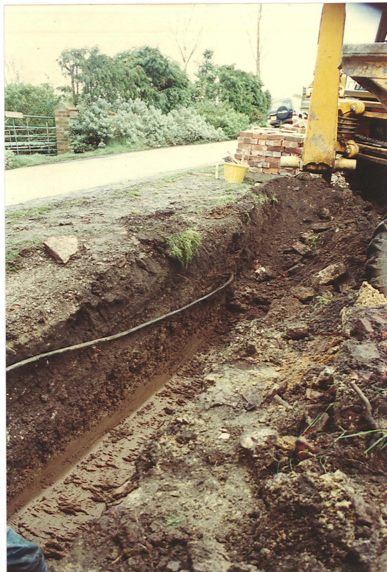
Pl. 6 Foundation trench with water pipe along road frontage, looking east
