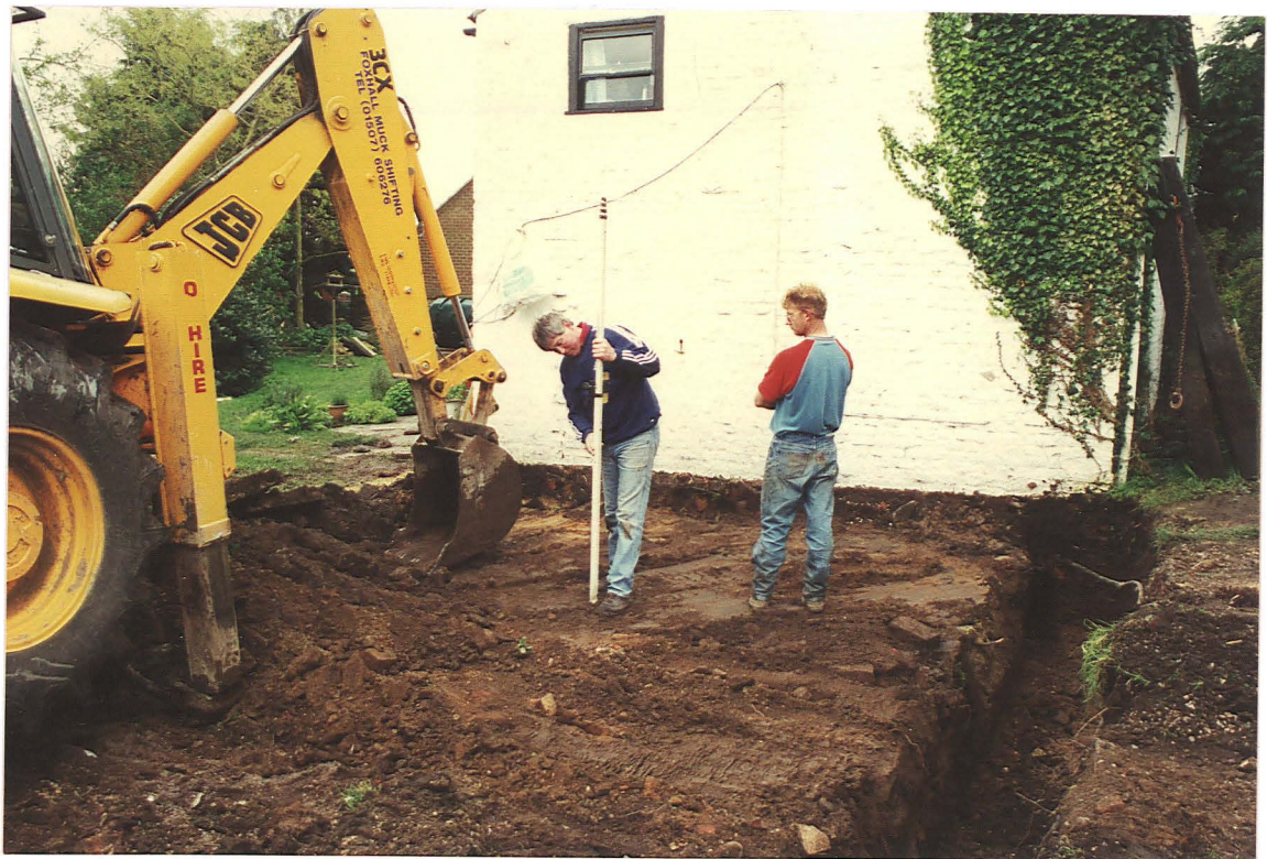
Pl. 4 Topsoil clearance in progress, looking west
