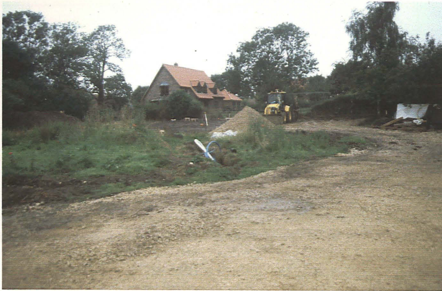
Plate 1 General view of development area during excavation, looking northwest
