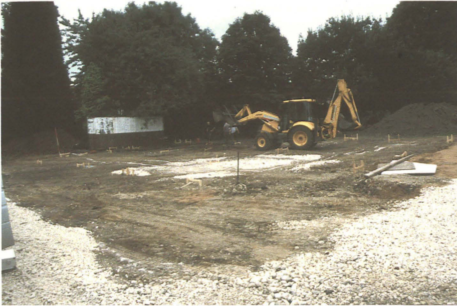
Plate 1 General view of development area during excavation, looking south
