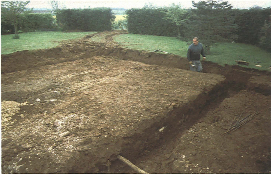
Plate 1 General view of development area during excavation, looking southwest
