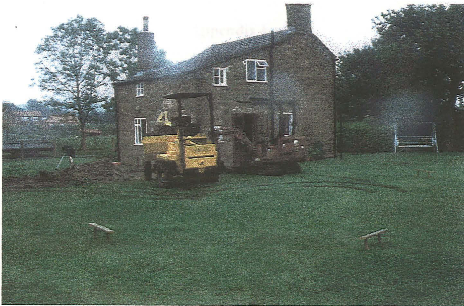
Plate 1 General view of site prior to groundworks, looking north east
