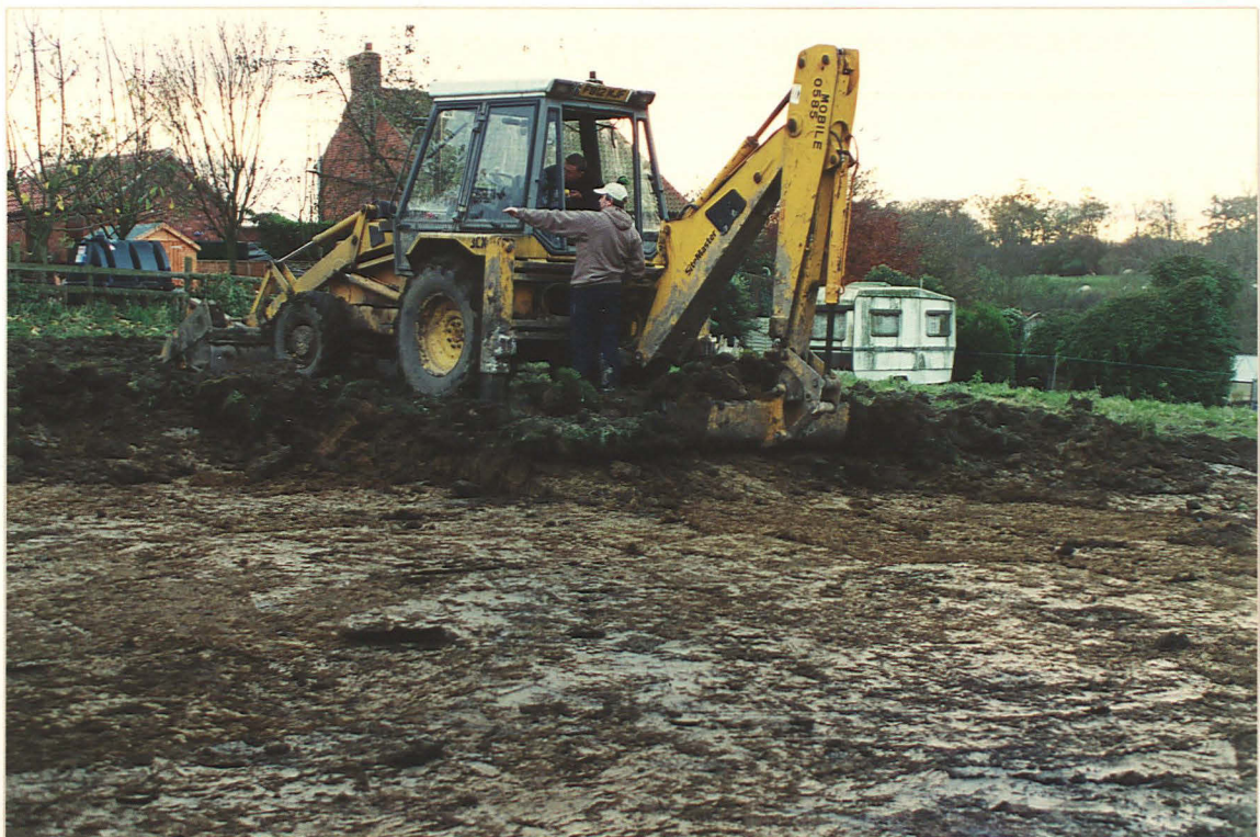
Pl. 4 Topsoil clearance in centre of site, looking south.
