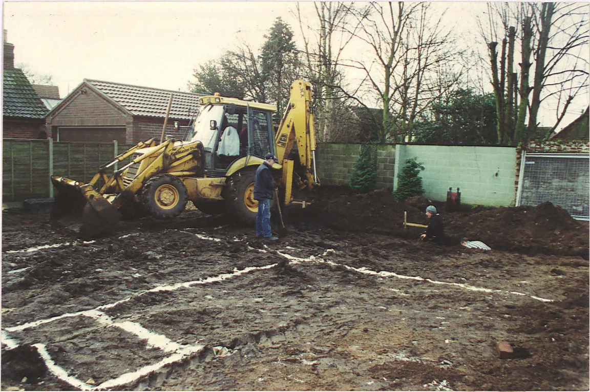
Pl. 1 Machine excavation of foundation trenches under archaeological supervision.
