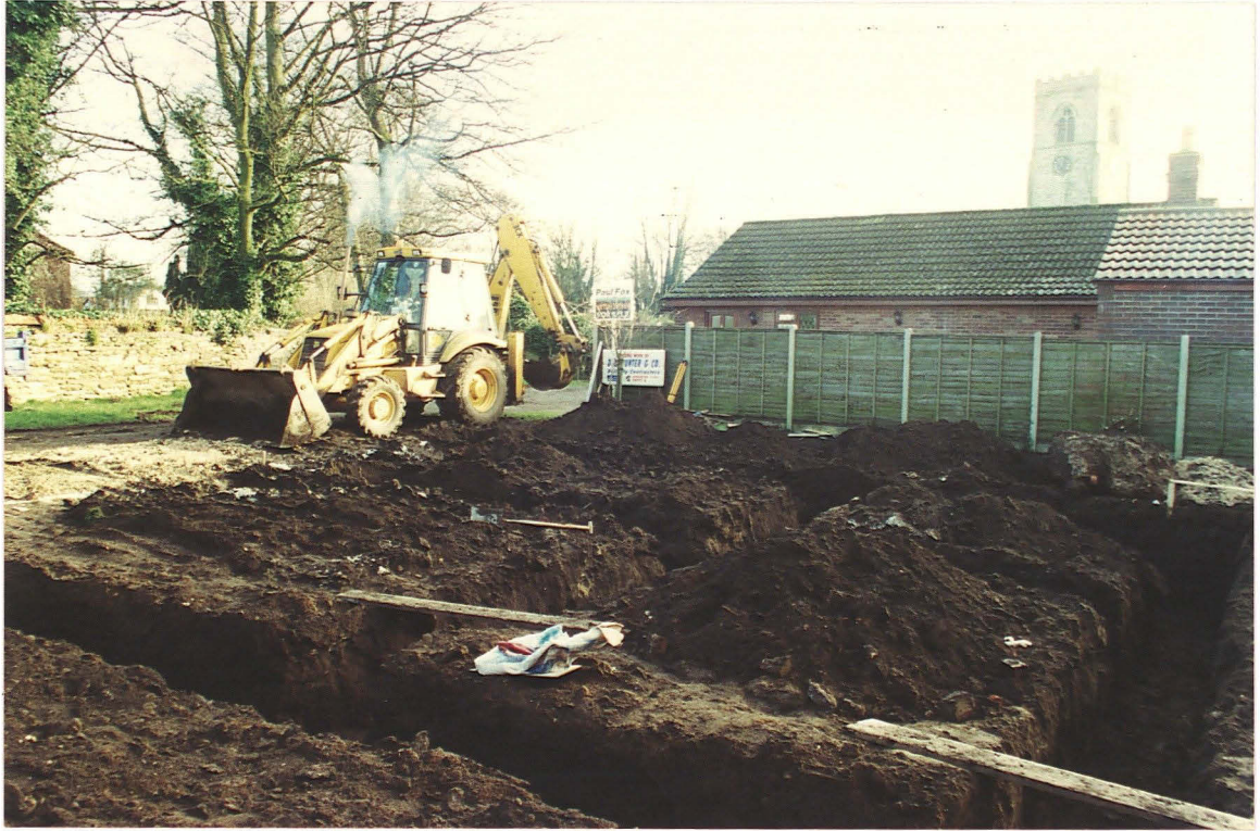
Pl. 3 The plot after excavation of trenches, looking east.
