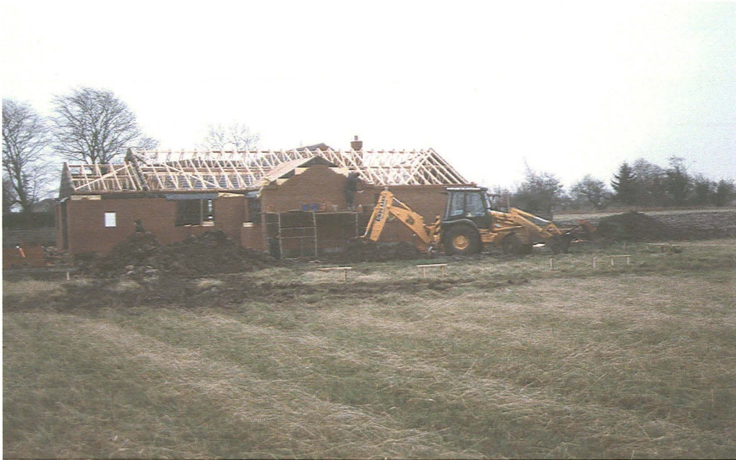
Plate 1 General view of site during groundworks
