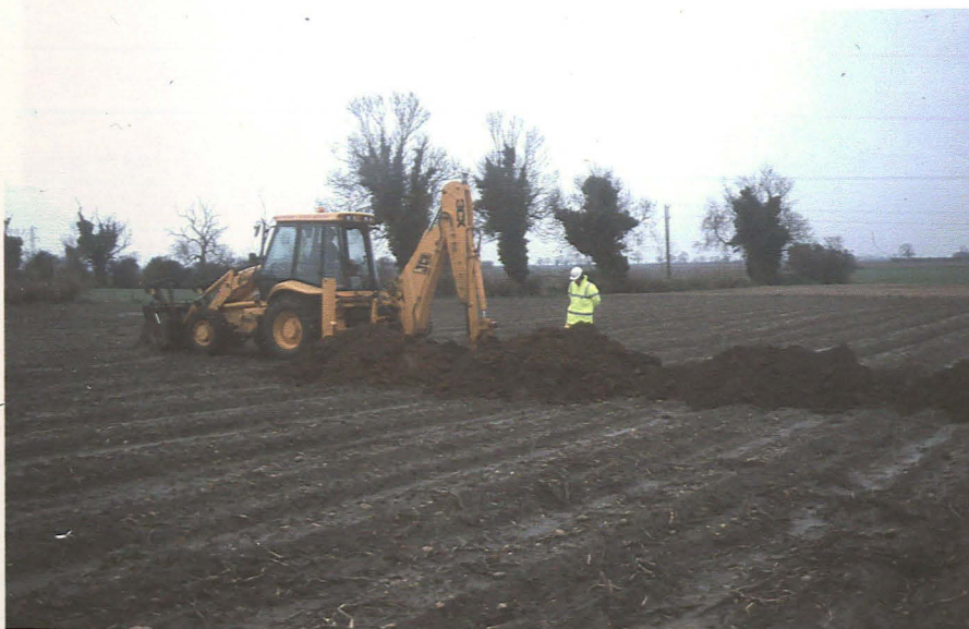
Plate 3 Machining of Trench 3 in progress, looking south
