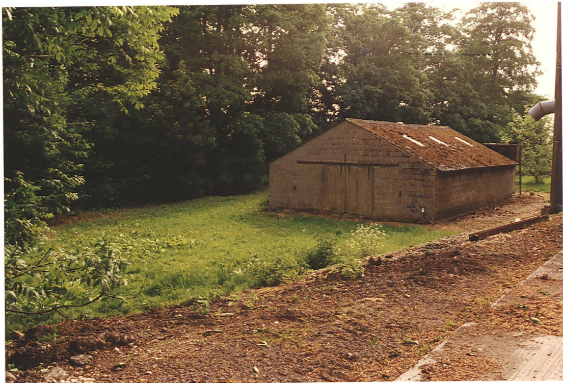
Pl. 3 Natural slope to north of existing grain store, used for tipping of excavated chalk (looking NE).
