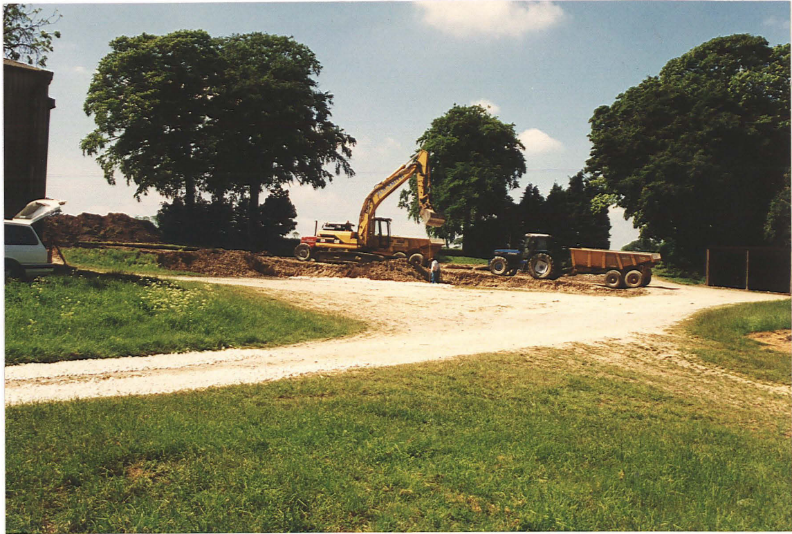
Pl. 2 Levelling the site after topsoil stripping (looking south across the farmyard).
