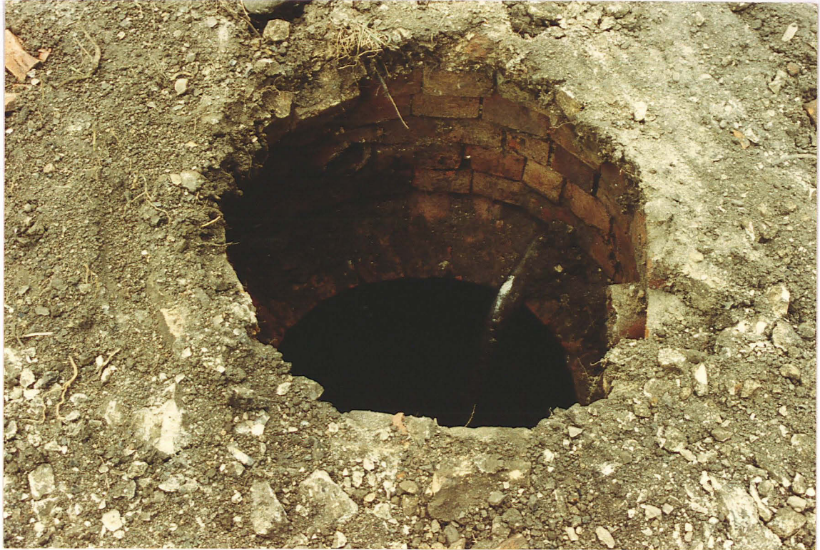
Pl. 14 Top brick courses of well 26, showing lead pipe.
