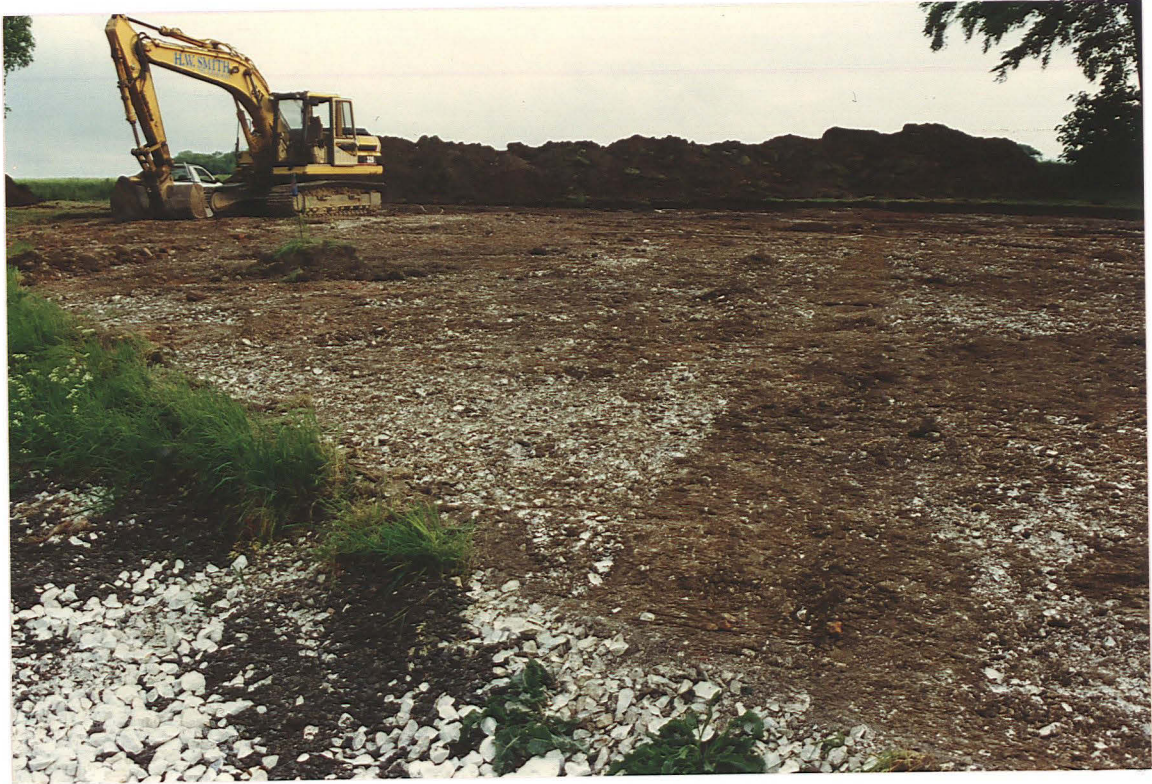
Pl. 4 Ditch 3 (linear, right) and pit 5 (right foreground, to right of the ditch). Brick rubble along the line of wall foundation 22 is visible, left background. Looking south.
