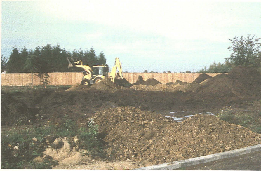
Plate 1 General view of site during groundworks.
