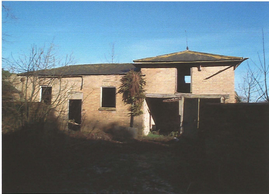
Plate 2 - The Stable Block, looking north
