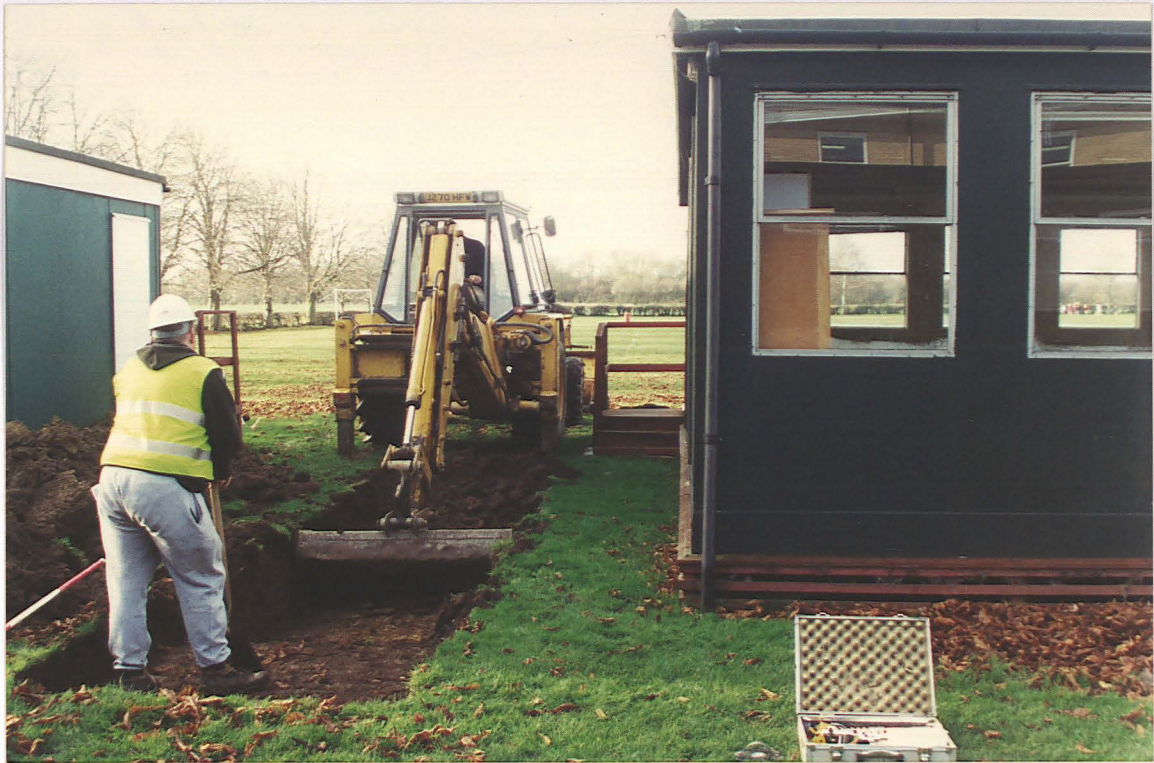
Pl. 1 Trench 1 during excavation
