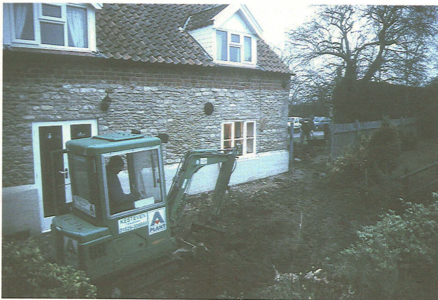
Plate 1 General view of site during groundworks.
