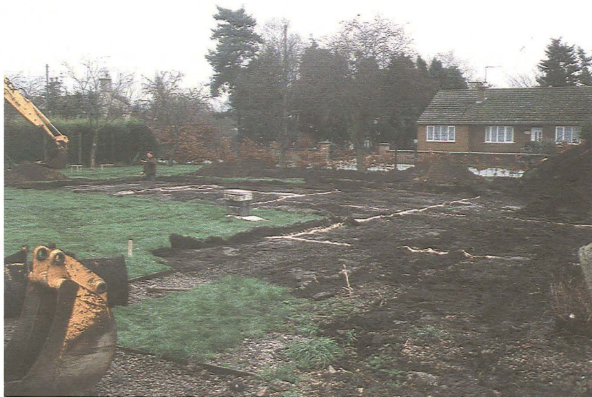
Plate 1 General view of site at start of groundworks, looking east
