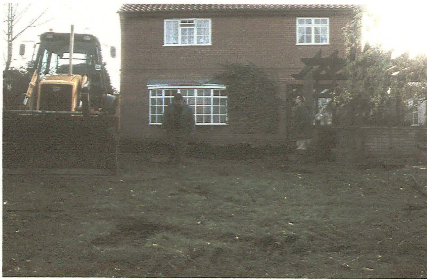
Plate 1 General view of site, looking south
