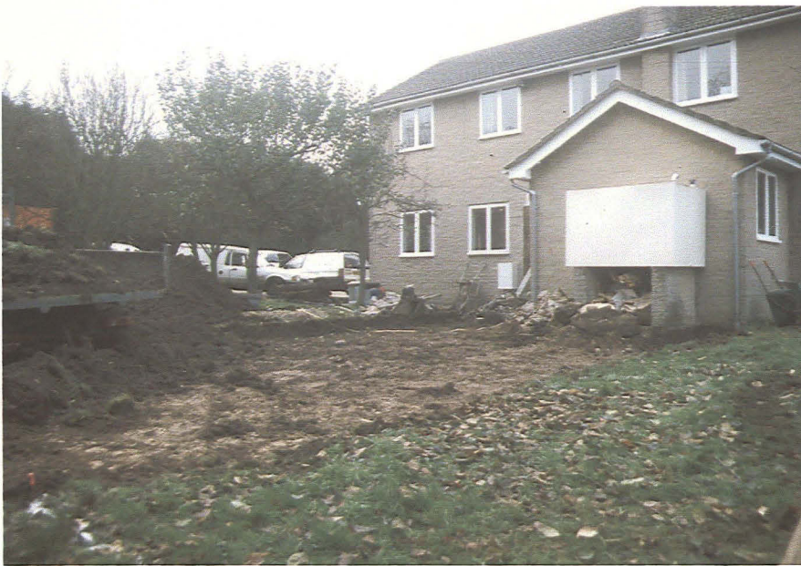
Plate 1 General view of site during site strip, looking northwest.
