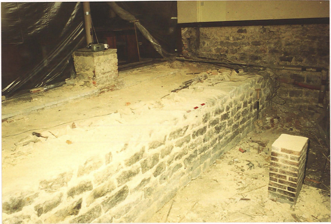
Pl. 7 Retaining wall 8, looking NW.
