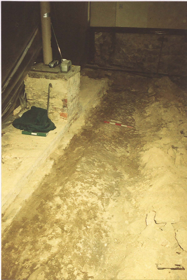
Pl. 5 Foundation trench 14 along north side of north aisle wall 1, showing stone foundation 2 . Looking west.
