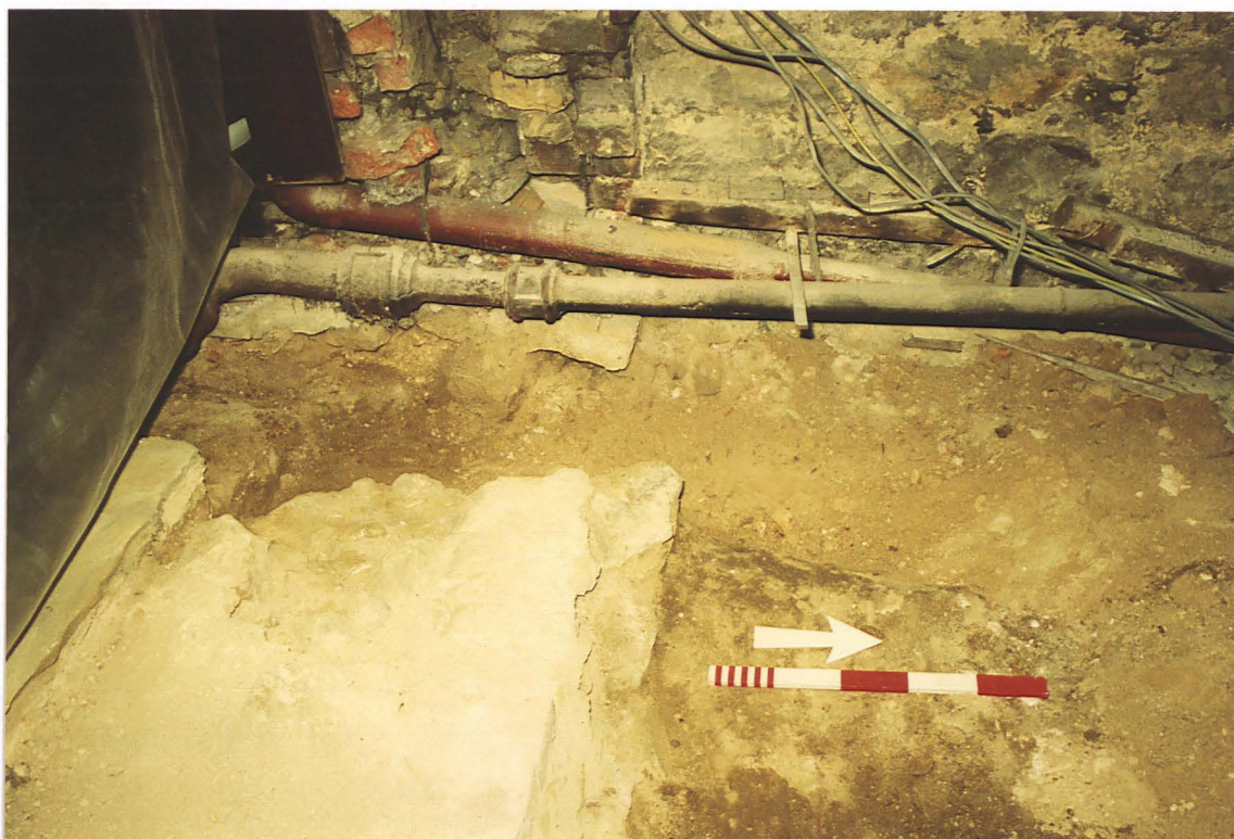
Pl. 6 Foundation trench 11 along north transept west wall. The trench cuts through the foundation of the demolished north aisle wall 1. Looking west.
