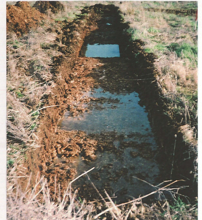
Plate 3: Looking north-east along trench 3
