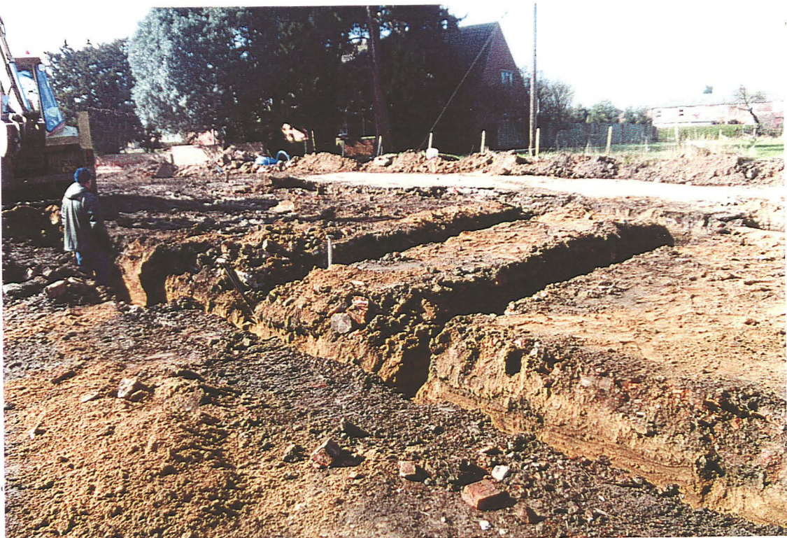
Plate 4: Shot of plot 4 foundations, looking south-west
