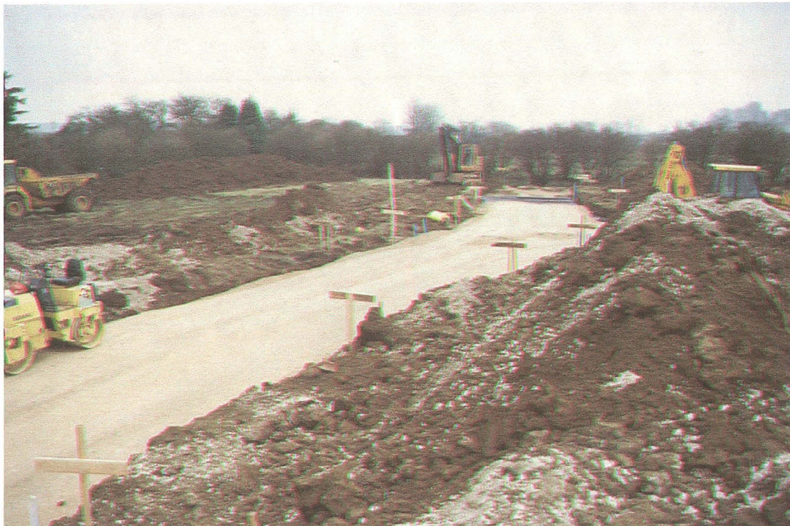
Plate 8: New access road after laying of hardcore sub-base - looking north
