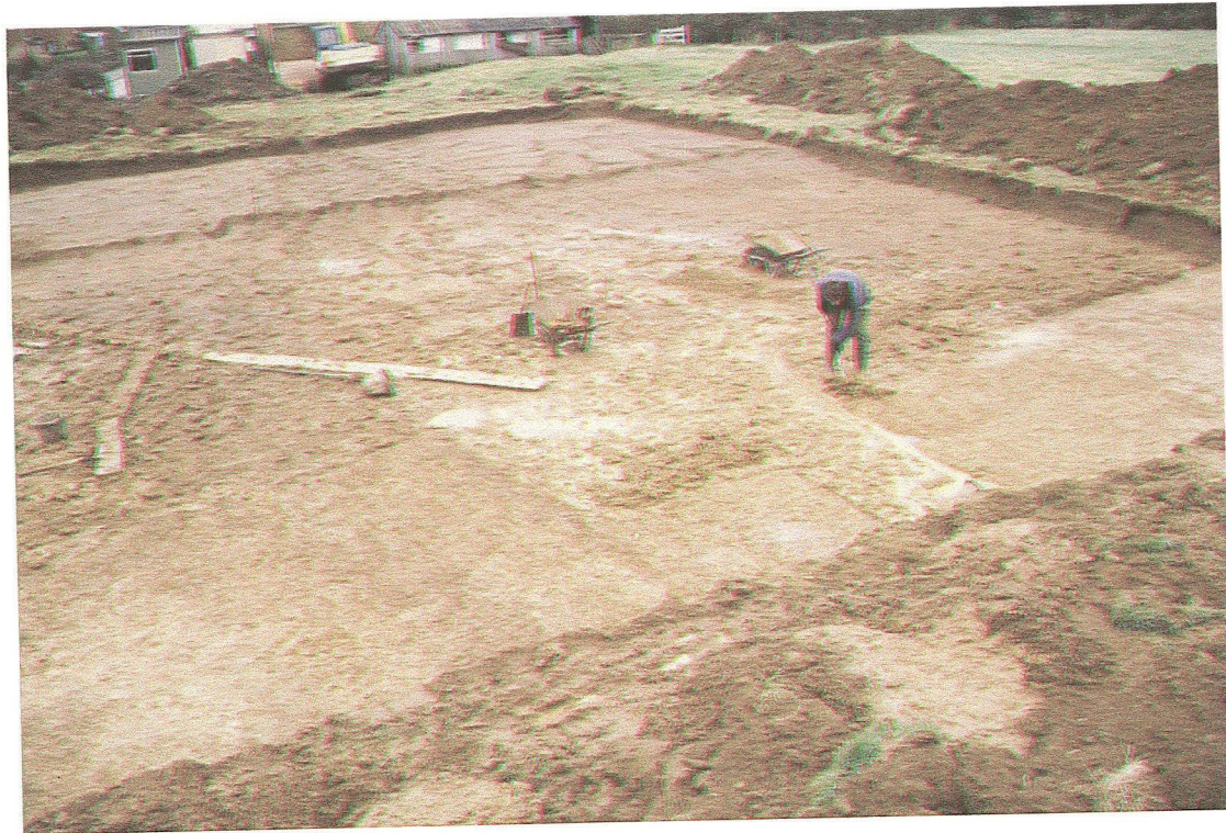
Plate 1: Initial cleaning underway, eastern end of Area 1 - looking north-west
