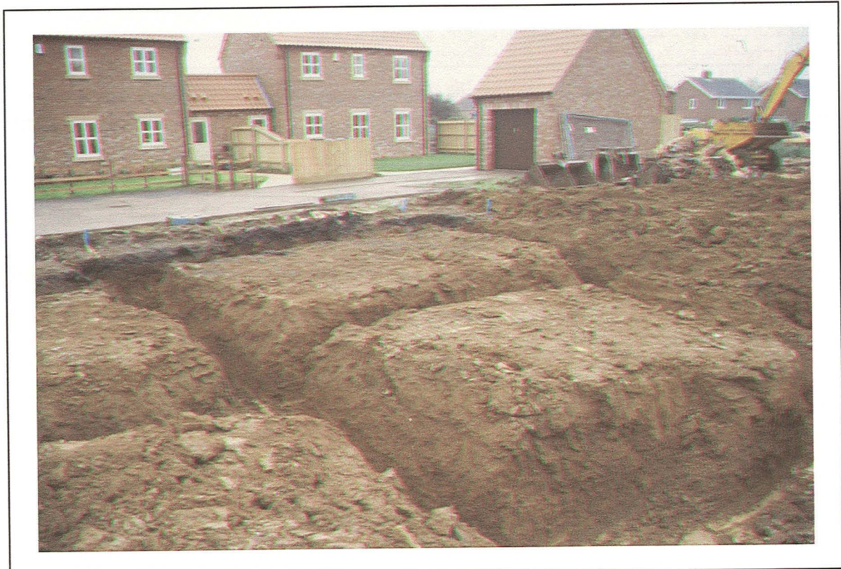
Plate 9: Overall view of Plot 4 - looking south-west
