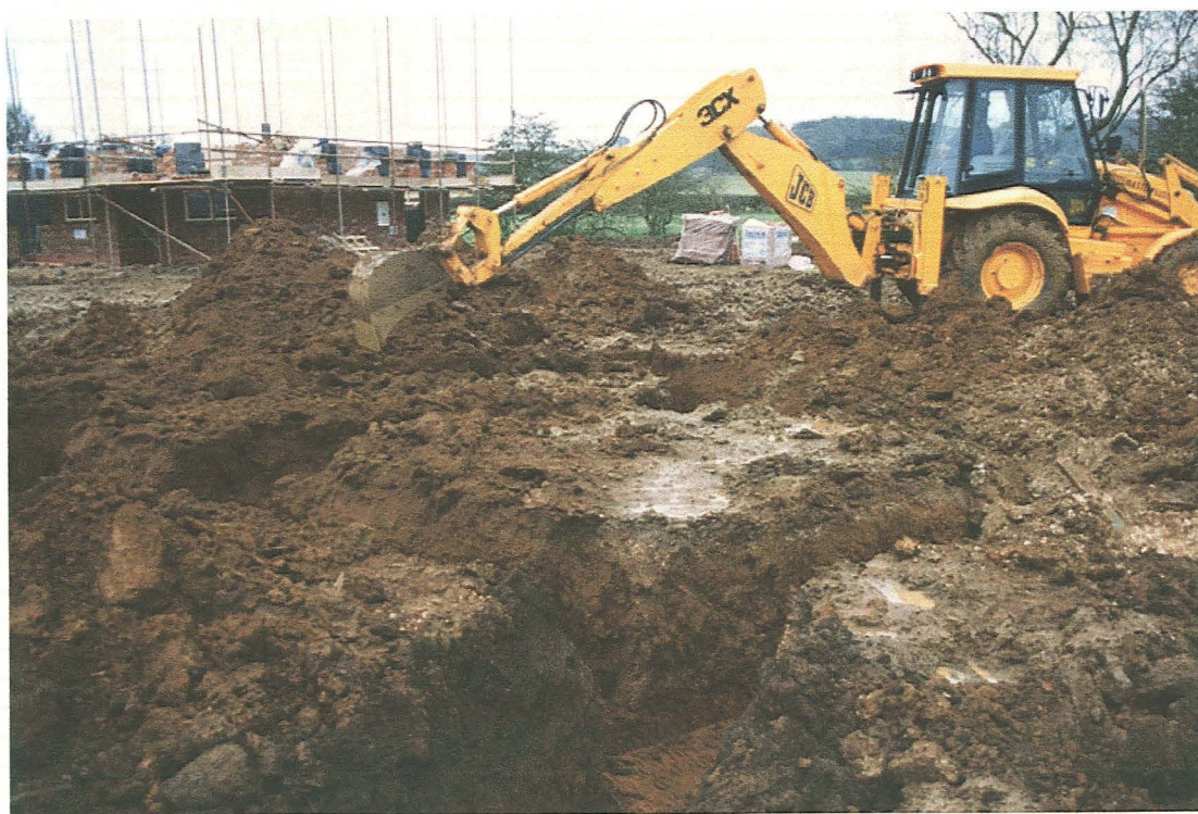
Plate 12: Excavation underway for Plot 8 - looking north-east
