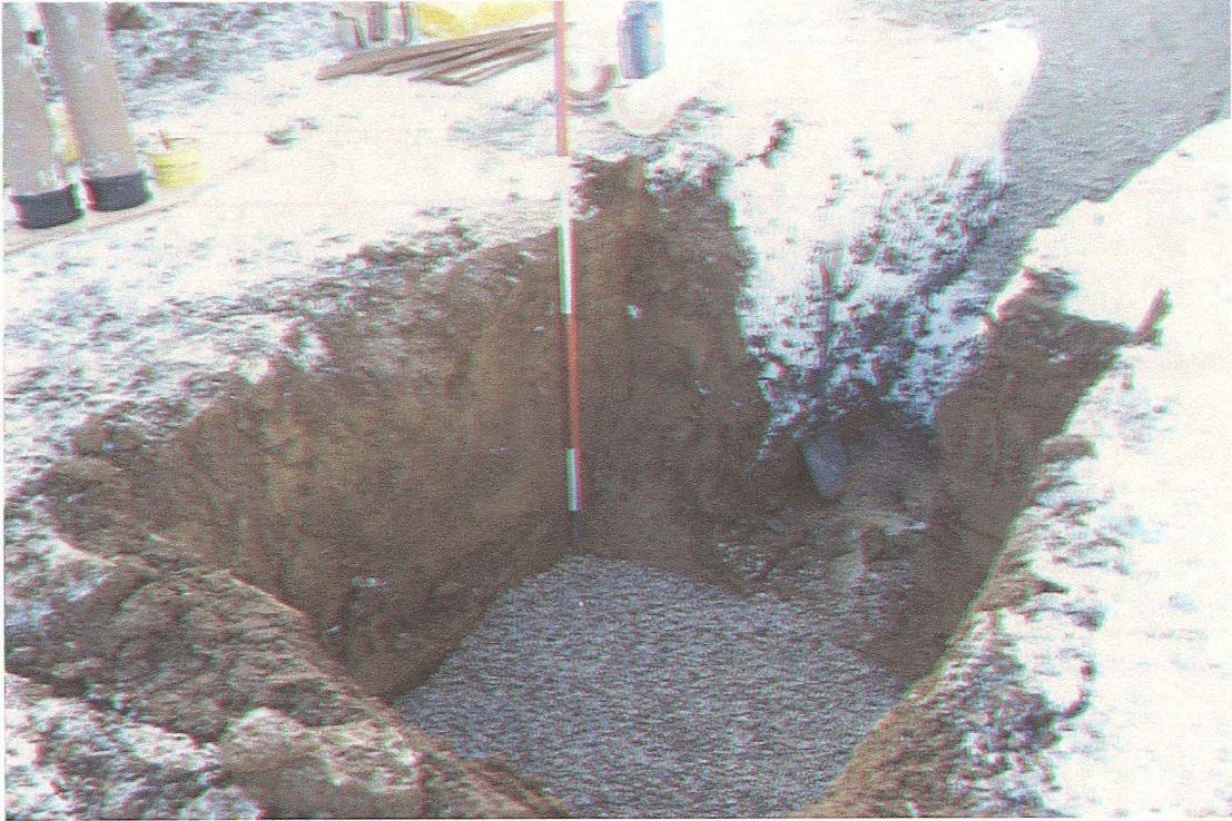
Plate 7: Trench for foul water sewer inspection chamber - looking south-east
