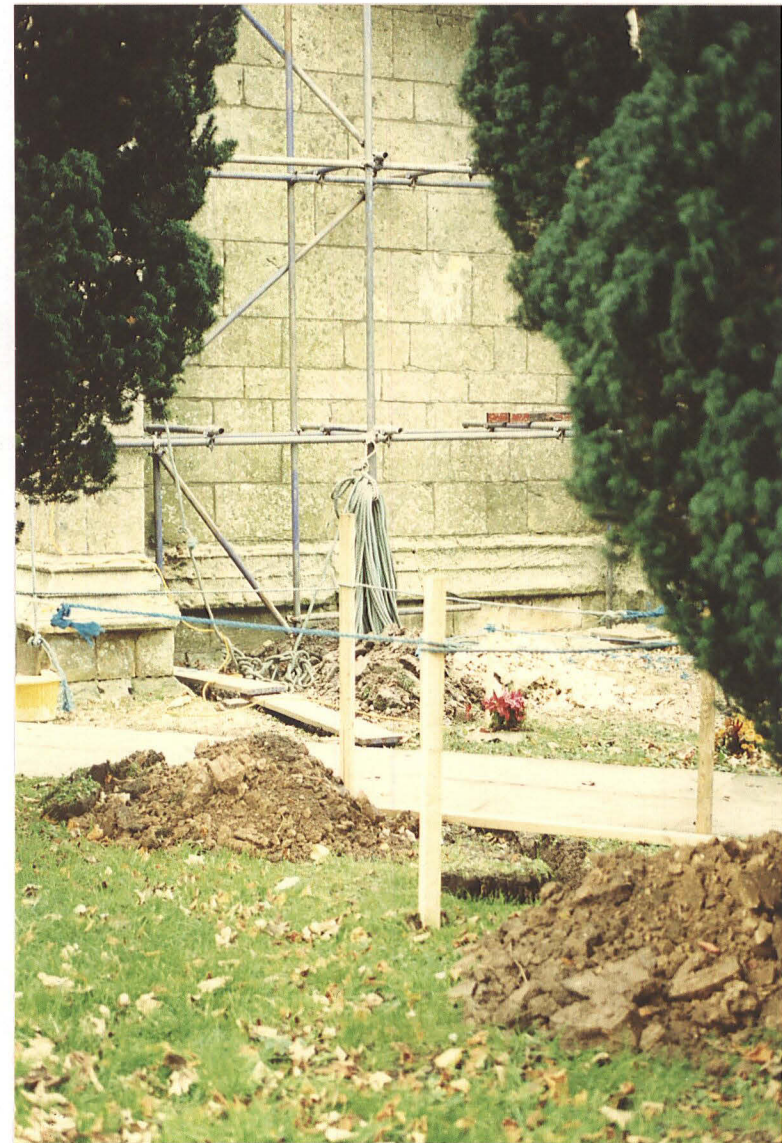
PI. 2 SW angle of the tower, showing scar left by removed rainwater pipe.
